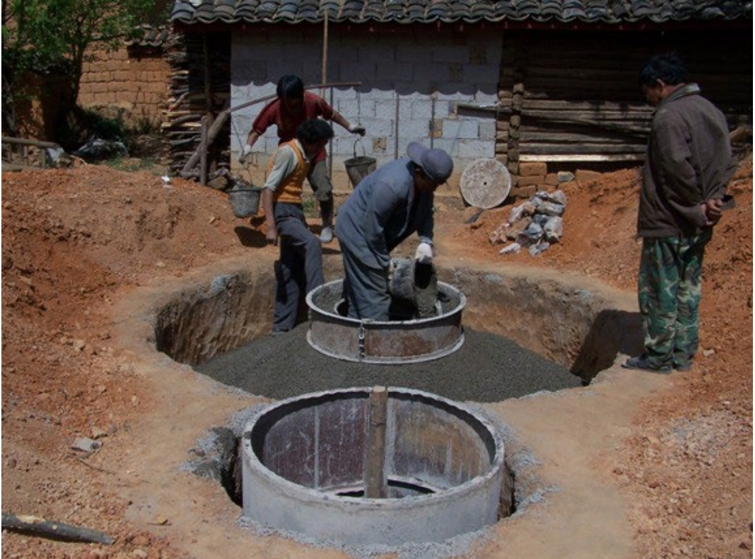
Figure 3. Domestic biogas digester under construction, Yunnan Province
