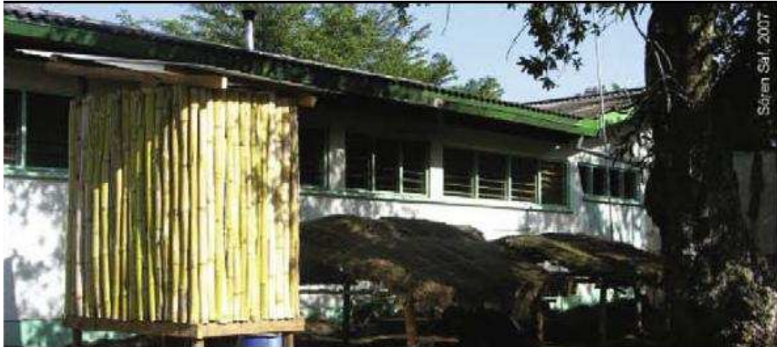
Figure 8: Outdoor Latrine/Digester Combination (Image Source: Martinssonb, Mboyya, Odhiamboa, Onyangoa & Sorenb, 2009)
