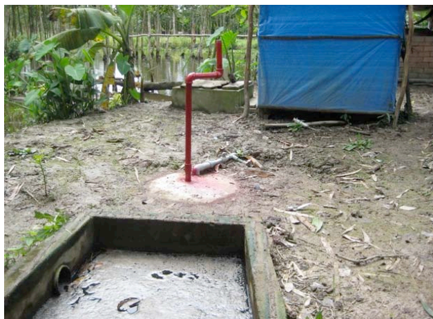
Figure 12. The completed EQ2 biogas plant with fulfilled outlet pit (left) and the crank handle installed inside digester with two blades (right) (Source: Nguyen and Do, 2009)
