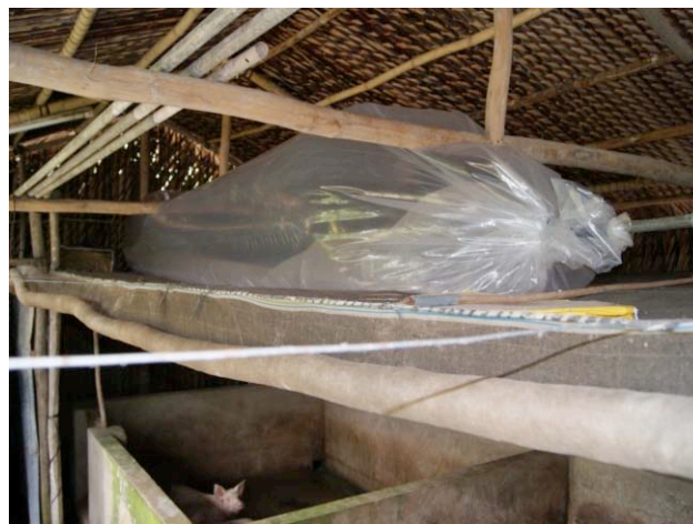
Figure 4. The digester body (left) and the gas-storage (right) of the PE model
