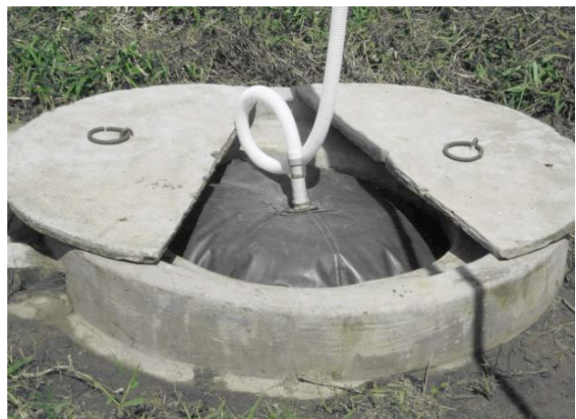
Figure 11. The HDPE top-layer with gas collection point (left) and the completed EQ1 plant with protect box and gas pipe (right)
