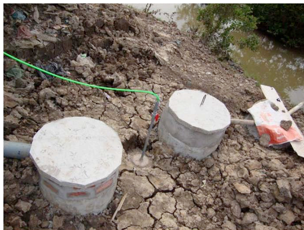
Figure 14. Installation of the composite digester (left) and after soil filled (right) (Photographer: Vo H. N.)
