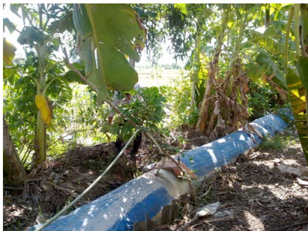
Figure 4. The digester body (left) and the gas-storage (right) of the PE model
