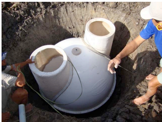
Figure 14. Installation of the composite digester (left) and after soil filled (right) (Photographer: Vo H. N.)
