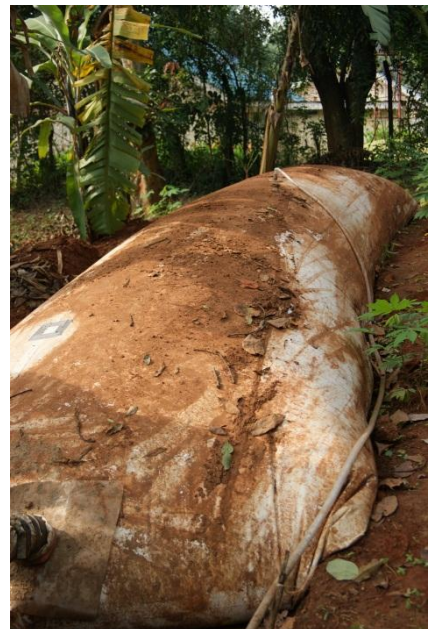
Figure 10 - Digester generating gas
