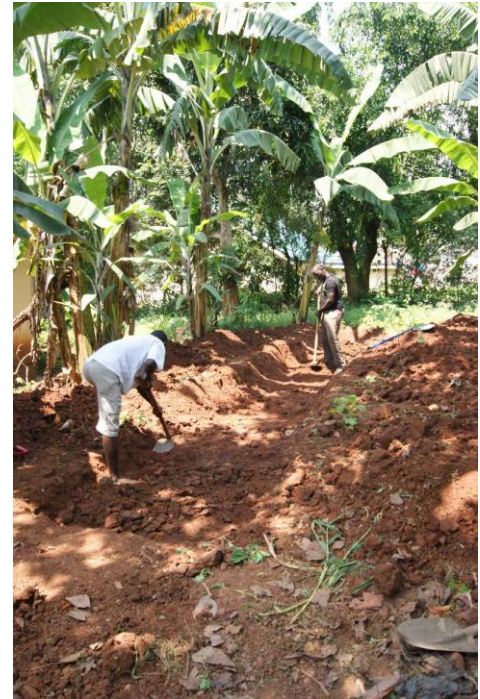
Figure 4 - Excavation of an 8m 3 digester ditch
