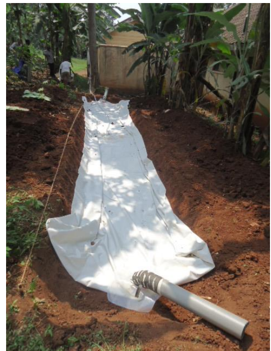
Figure 6- Digester bedded into the ditch
