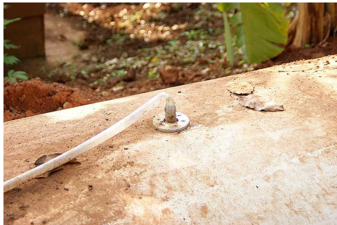
Figure 11 – Potential problem - bend in gas line leading to blockage
