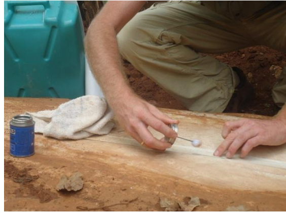
Figure 8 - Glue applied to fix the digester
