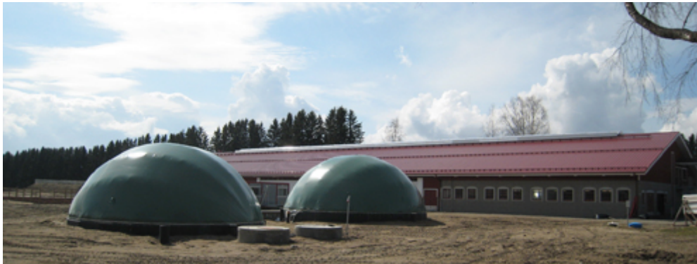
Figure 4. Research and training plant of Maaninka. Digester is 300 m 3 . The plant includes also a second stage digester of 300 m 3 . For research the temperature of digester can be varied between 20-55 deg. C. The usual temperature is 37 deg. C. About 80 kW of heat and 50 kW of decentralised electricity are produced with a high efficiency gas motor. Manure of 100 cows and different agricultural products are used as raw materials. (source: https://portal.mtt.fi/portal/page/portal/mtt/mtt/tutkimus/infrastruktuuri/maaningangutkimusalusta ).
