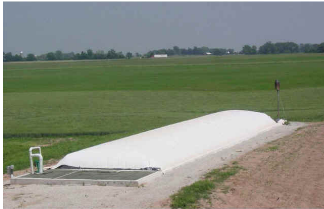
Figure 6: Stencil Dairy plug flow digester for 1200 cows
