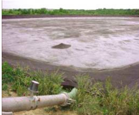
Figure 4: Example of anaerobic covered lagoon and biogas recovery
