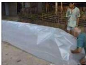
Photo 29. Pumping air until the tube is full
