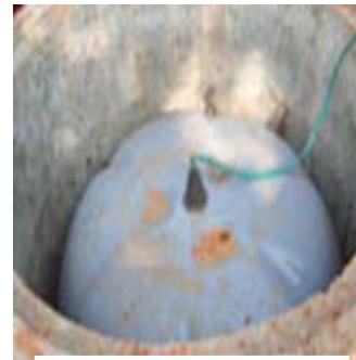
Fig. 3i. Installation of gas holder
