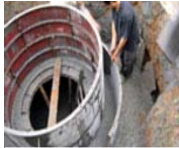
Fig. 3e. Assemble the digester mould (IInd day)
