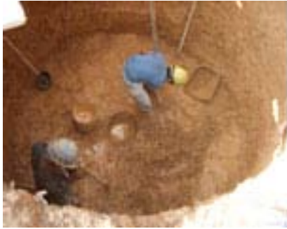
Fig. 3a. Dig a hole in the ground (1st day)
