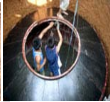
Fig. 3c. Assemble the upper part of mould (1st day)
