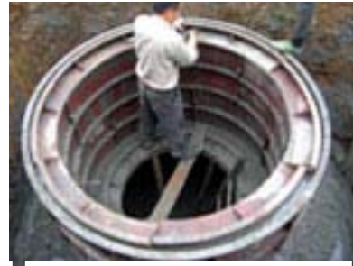
Fig. 3f. Casting the digester (IInd day)
