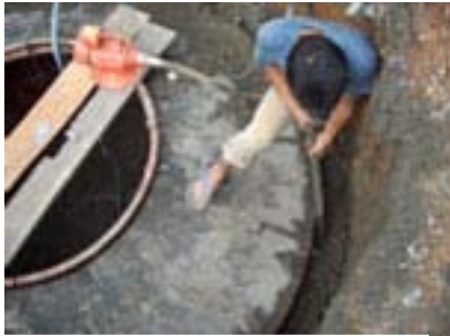
Fig. 3d. Casting the digester (IInd day)
