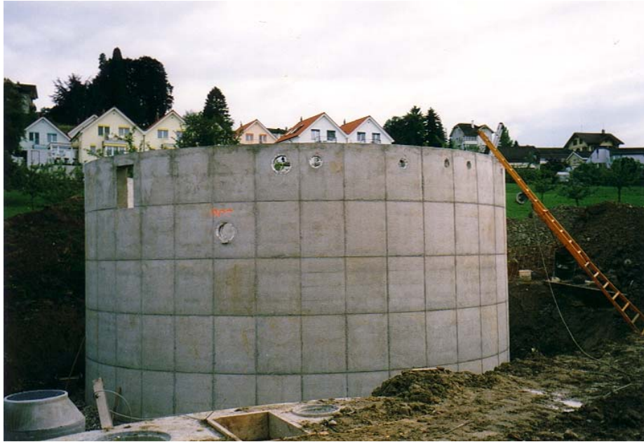
Figure 5: Outside Walls of digester with necessary clearances
