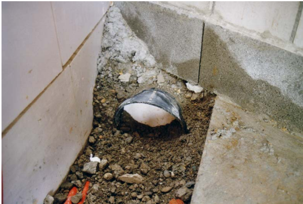
Figure A12: Compact biogas plant "Flach": Spare pipe machine room
