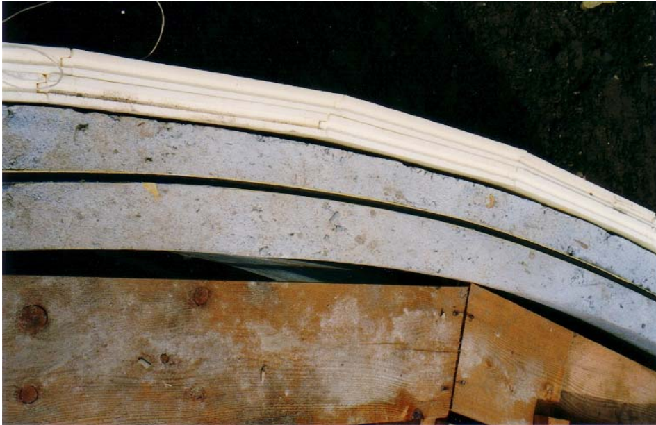
Figure 19: Wall composition of digester
