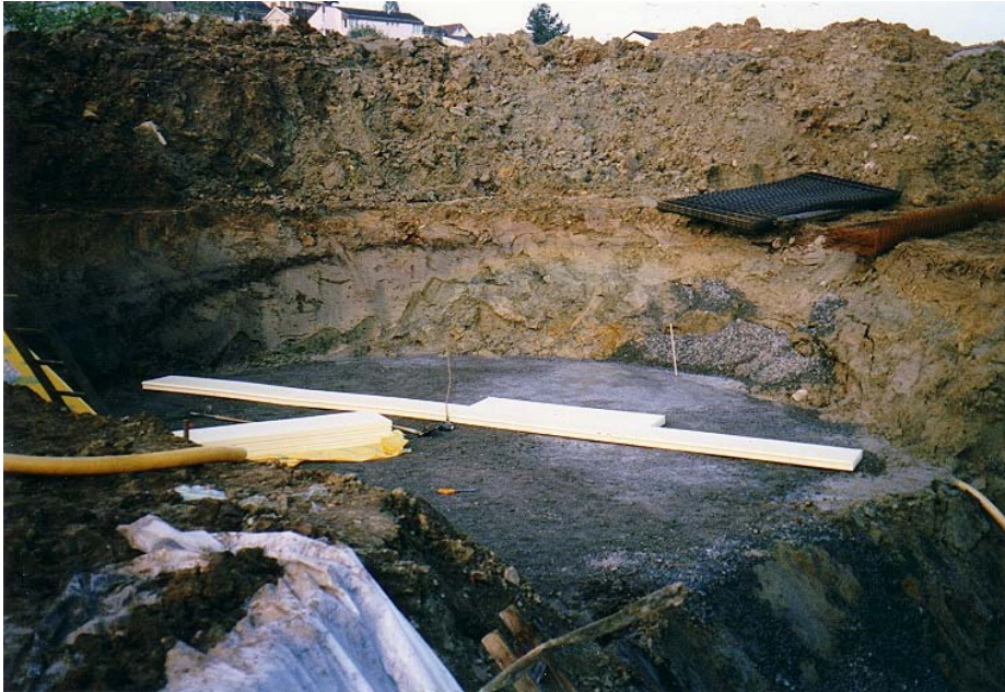
Figure 1: Ground leveling and begin of floor insulation
