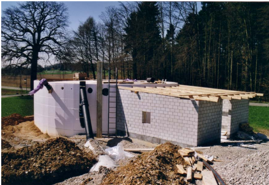
Figure A2: Compact biogas plant “Flach”: Outside View
