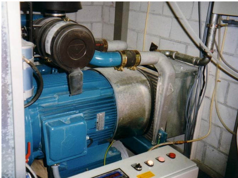
Figure 18: Electric generator of cogeneration unit
