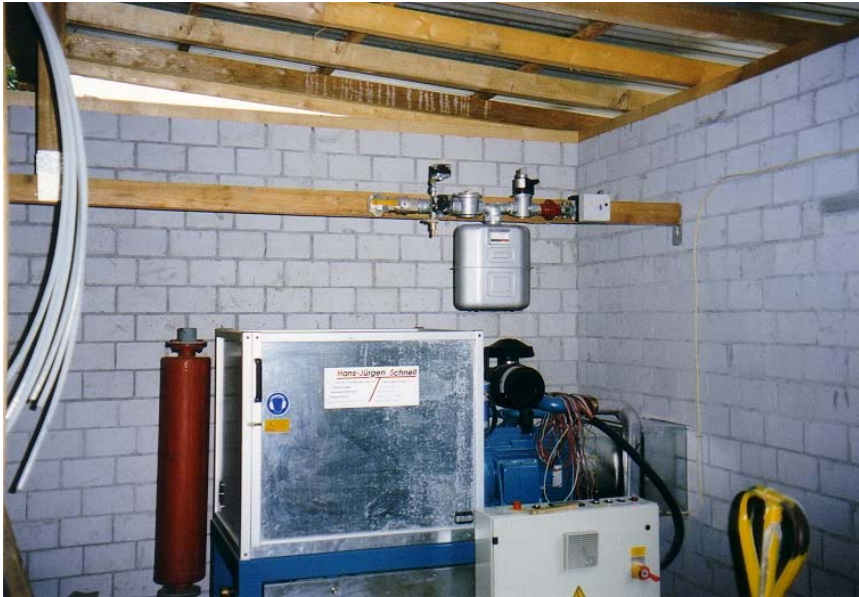
Figure 11: Positioning cogeneration unit
