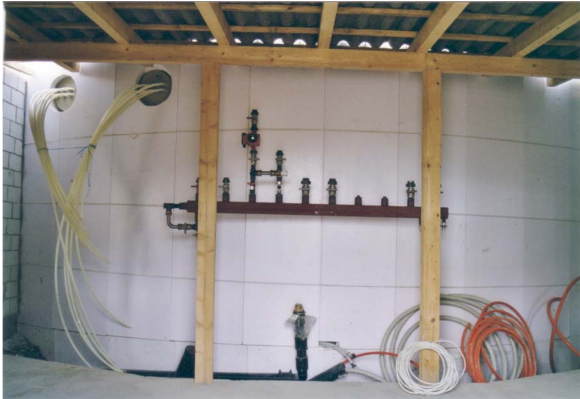
Figure A1: Compact biogas plant “Flach”: Inside machine room
