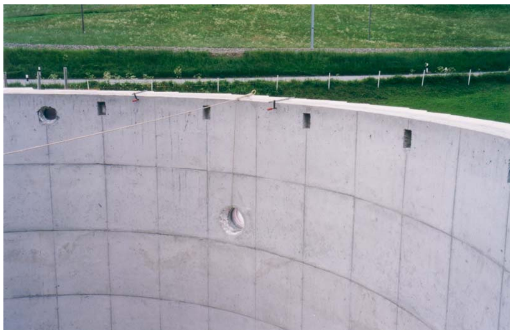
Figure A4: Compact biogas plant “Grass”: Inside digester view
