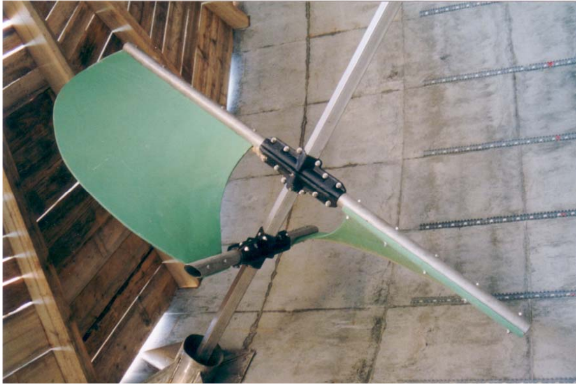
Figure A9: Compact biogas plant “Flach”: Agitator
