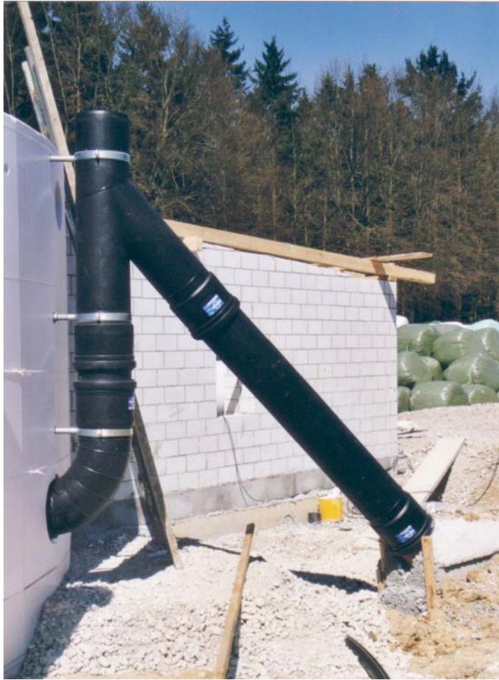
Figure A11: Compact biogas plant "Flach": Spillway digester
