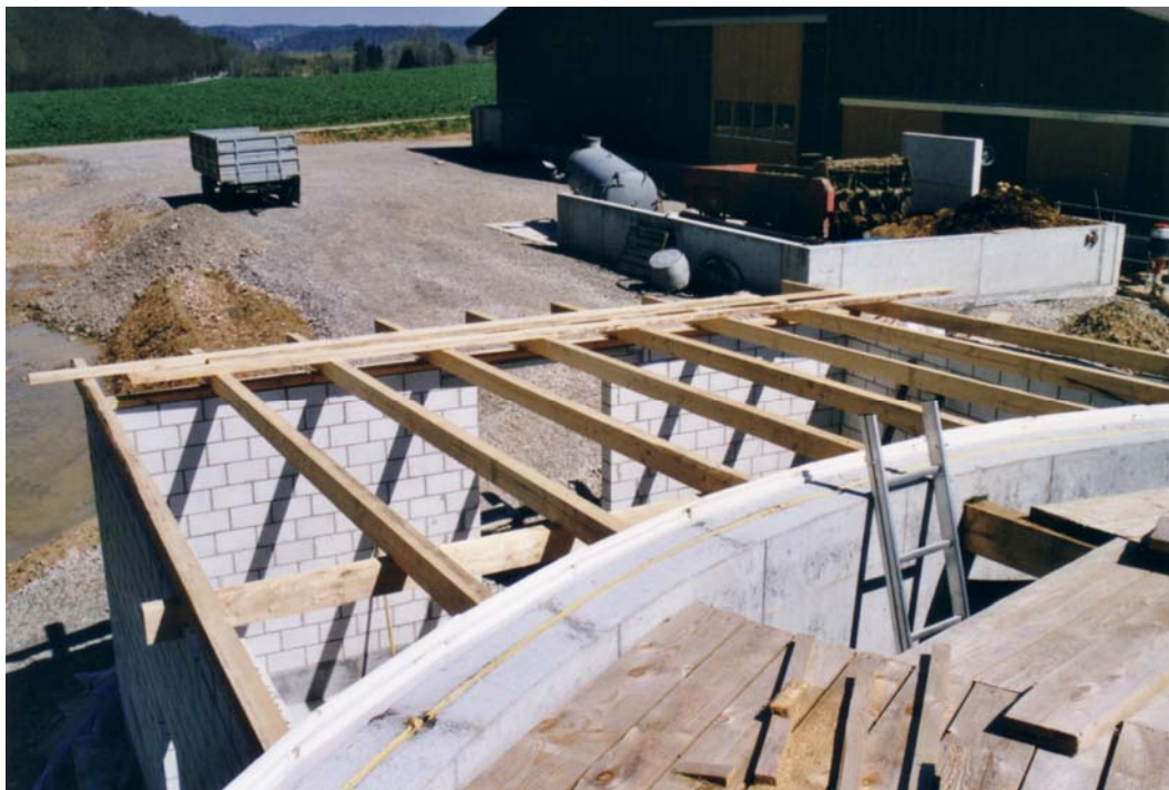
Figure A6: Compact biogas plant “Flach”: Machine room from on top
