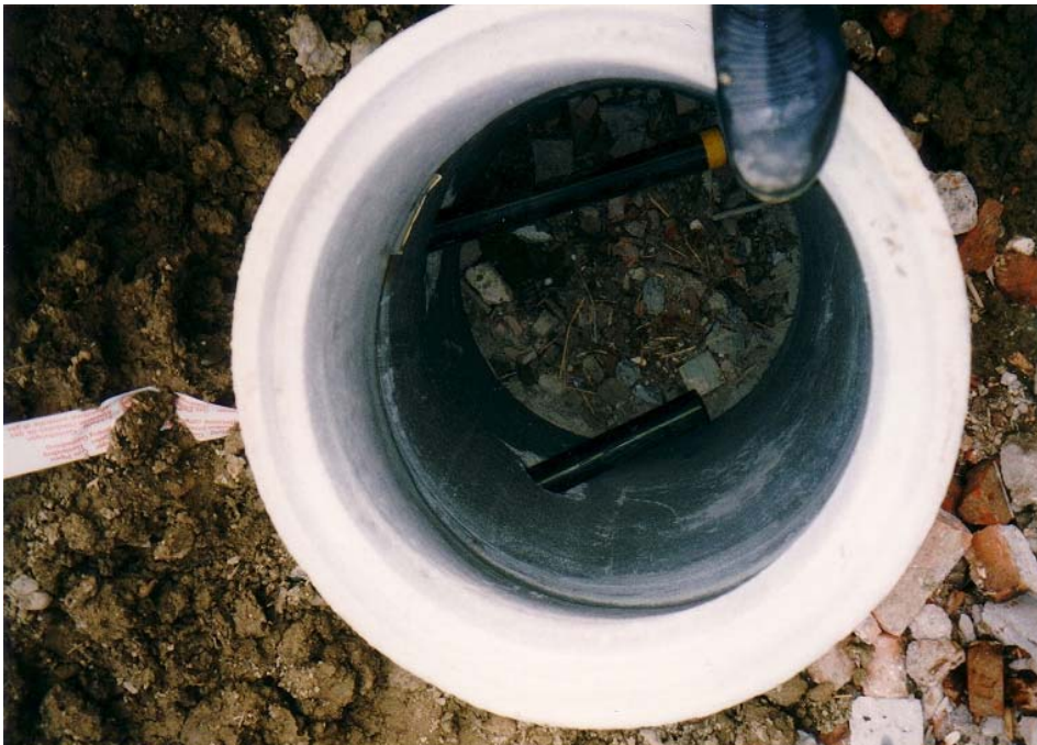
Figure 20: Control duct with condensate trap
