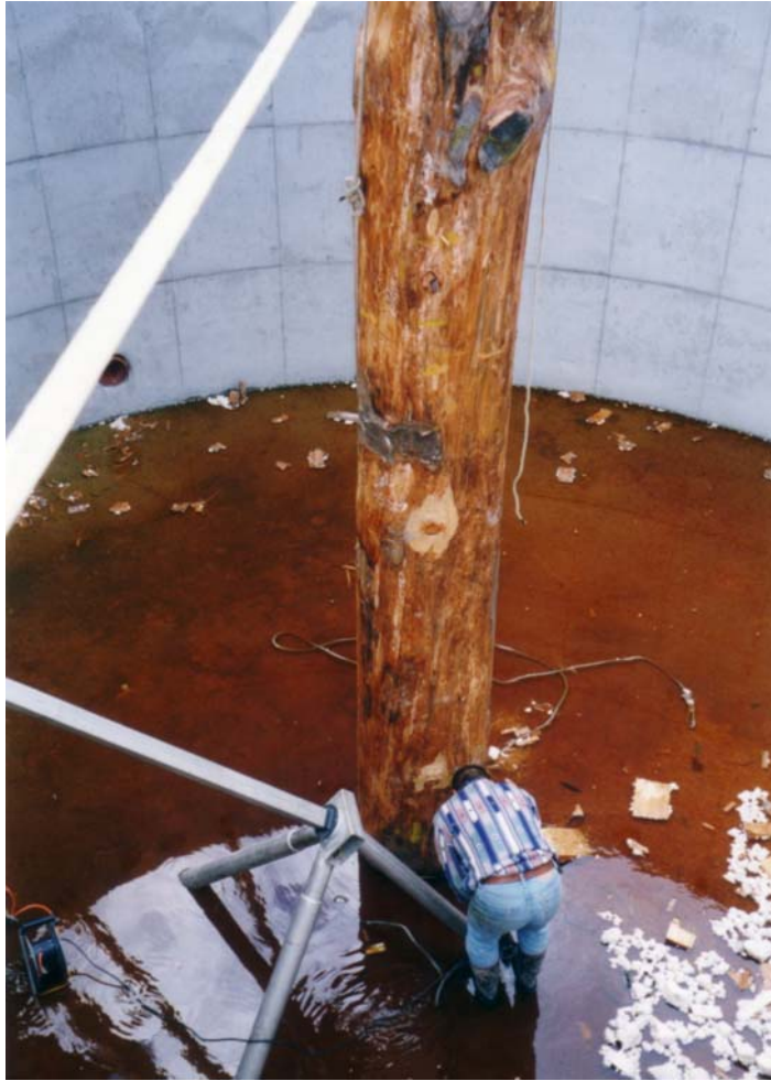
Figure A4: Compact biogas plant “Grass”: Middle post
