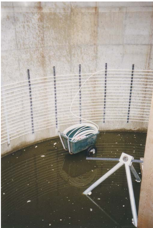
Figure 8: Wall heating of digester and bottom bearing-stand of agitator
