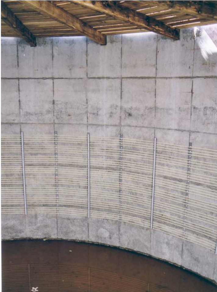
Figure A5: Compact biogas plant “Flach”: Digester heating
