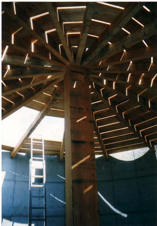
Figure 10: Digester wooden top (interior view)
