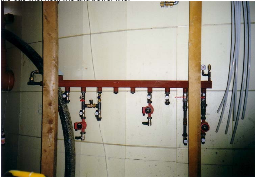
Figure 12: Premounted heating distributor
