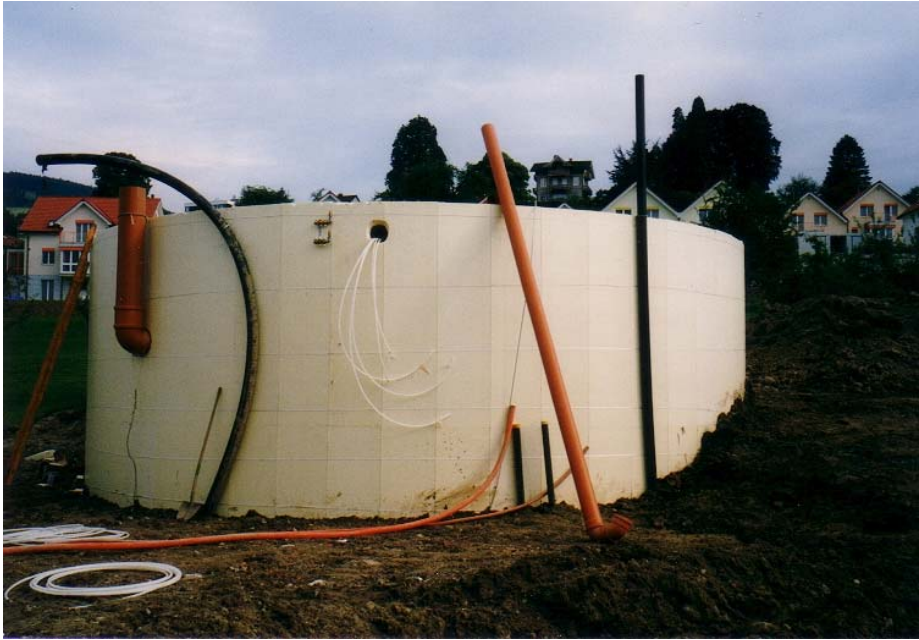
Figure 7: Finished Wall insulation with supply lines
