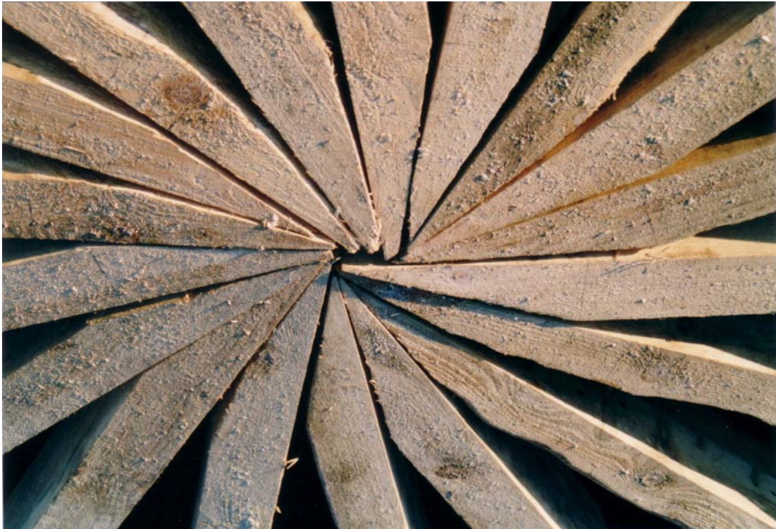
Figure A10: Compact biogas plant “Flach”: Wooden top support beams
