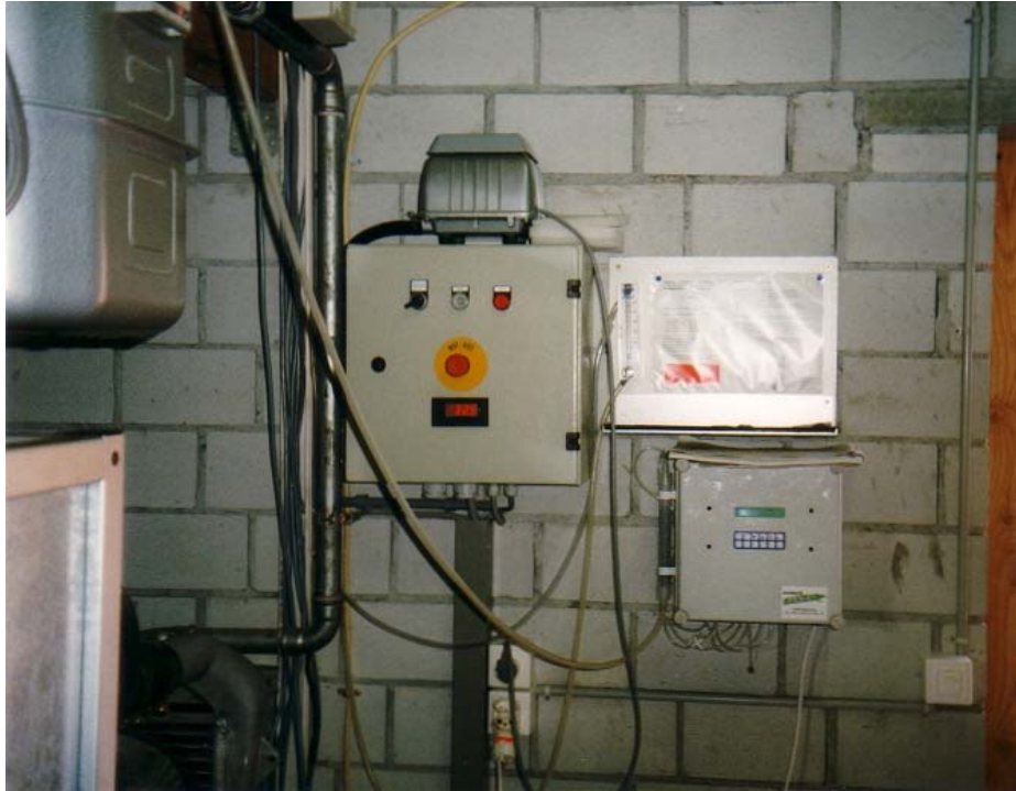
Figure 13: Agitator control cabinet, sulfur and methane gauge
