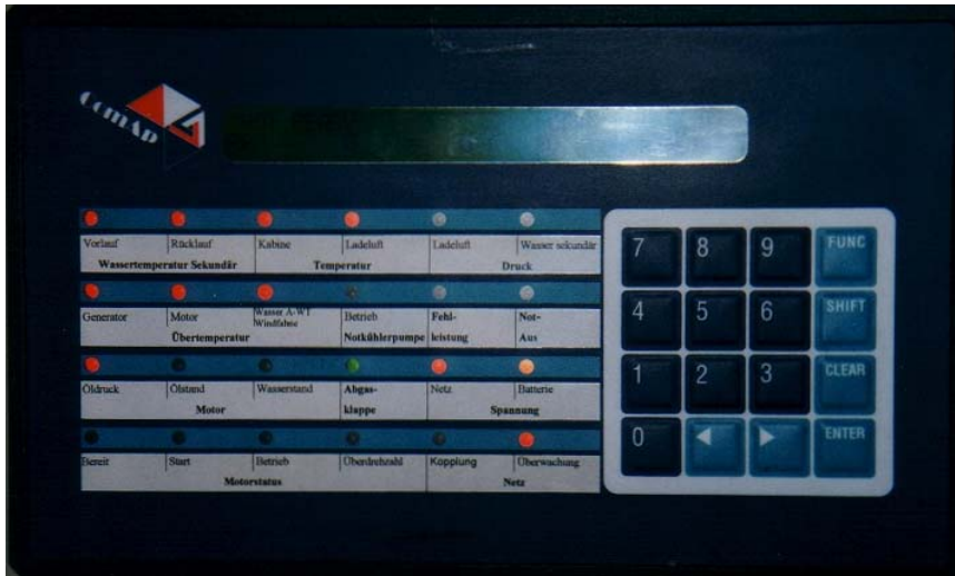
Figure 14: Display of the cogeneration control unit
