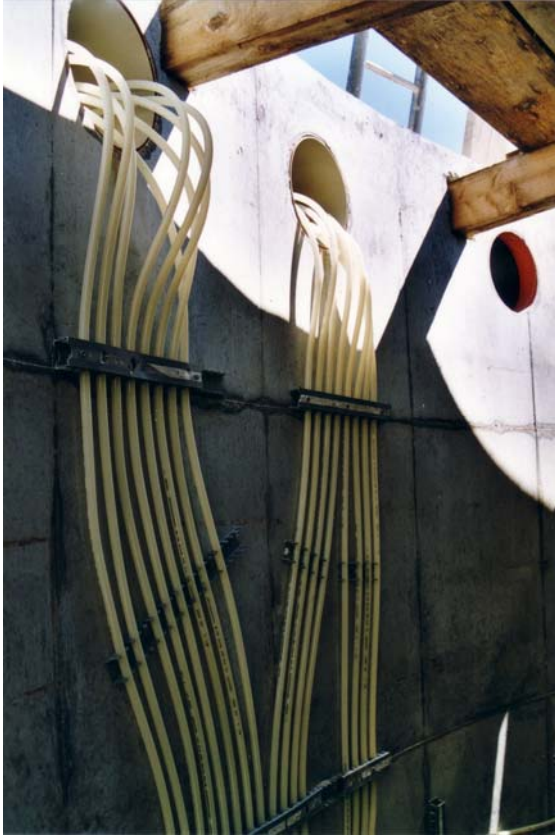
Figure A7: Compact biogas plant “Flach”: Digester heating
