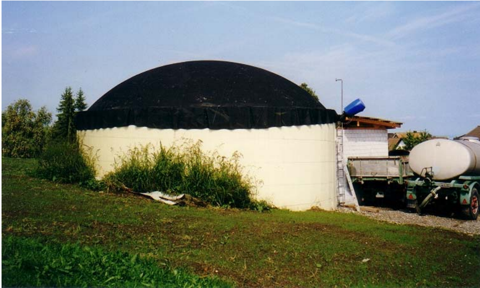
Figure 21: Digester without wooden casing
