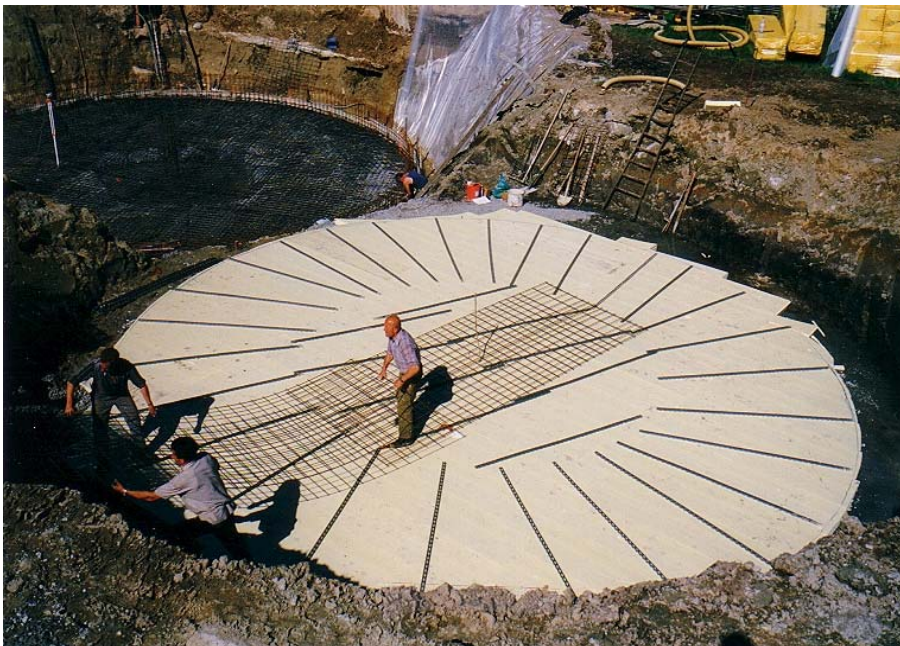
Figure 2: Bottom insulation
