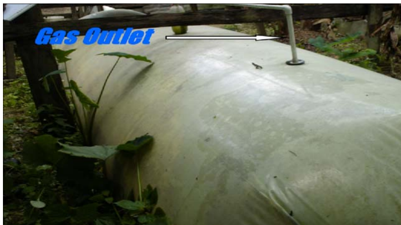
Fig.7 Completed gas outlet
