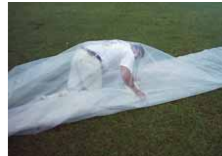
Above: Threading bio-digester bags. Be careful not to tear the bags.
