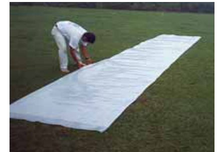
Above: Threading bio-digester bags. Be careful not to tear the bags.
