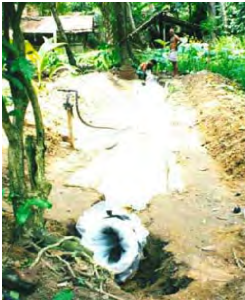
Figure 12. When water reaches the level of buckets, both ends are opened. Water level keep gases inside the bag, forming a bell.
