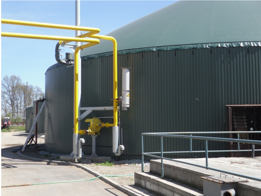
Figure 39: Start of biogas pipes to a satellite CHP unit to the town of Trebon, Czech Republic (Source: D. Rutz)
