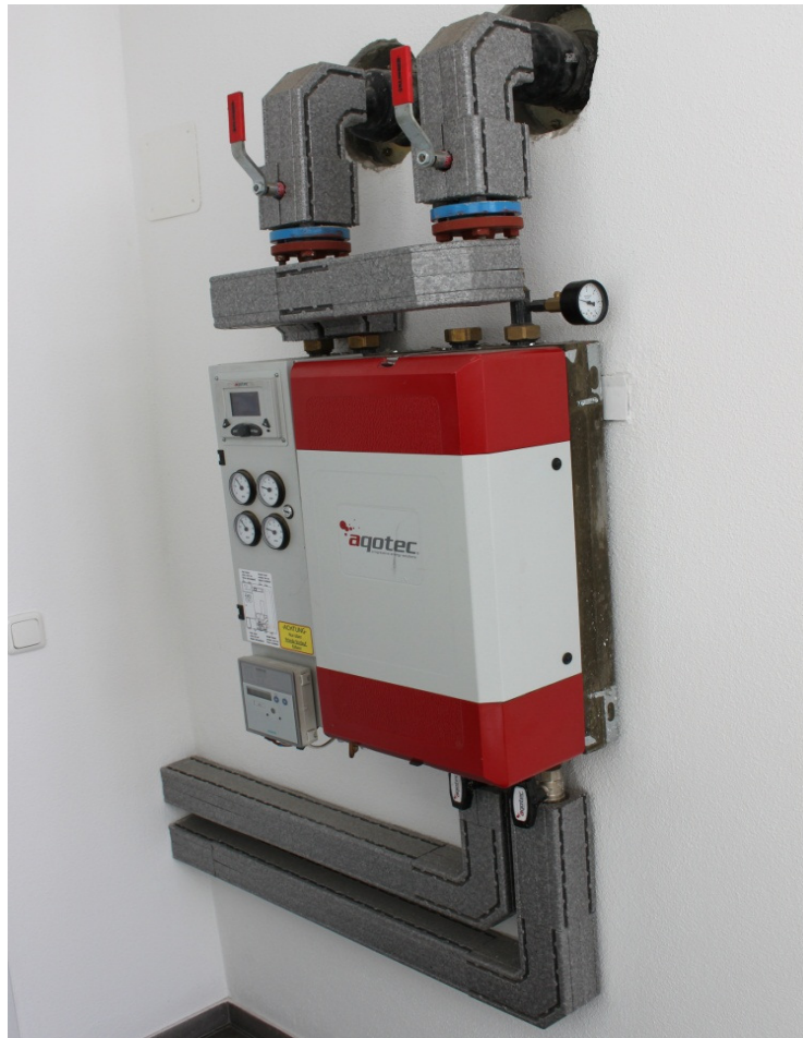
Figure 11: Connection equipment (including a heat exchanger) of an end consumer connected to a district heating system in Achenal, Germany (Source: Rutz)
