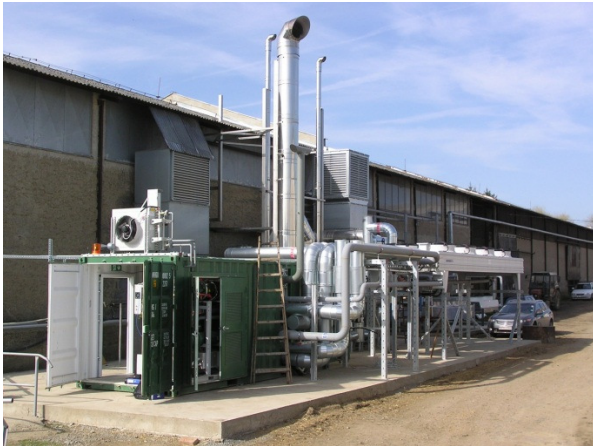
Figure 32: ORC system (using R245fa) of a biogas plant in Dublovice, Czech Republic (Source: GE Energy)
