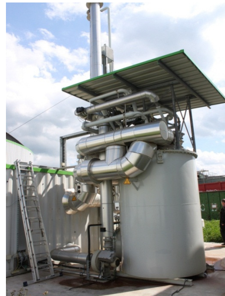
Figure 4: Low calorific value (LCV) burner of a biogas upgrading plant for digester heating in Aiterhofen, Germany (Source: Rutz)
