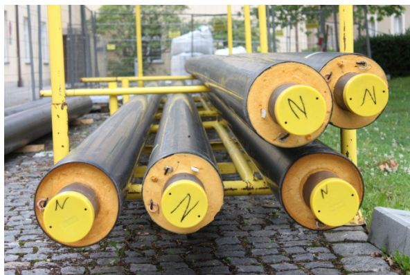
Figure 13: Insulated pipes for district heating in Germany (Source: Rutz)
