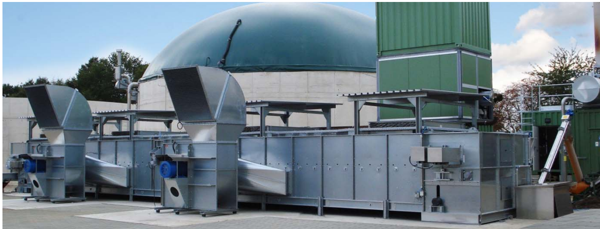
Figure 25: Belt dryer for digestate drying in front of a biogas plant (Source: STELA Laxhuber GmbH)
