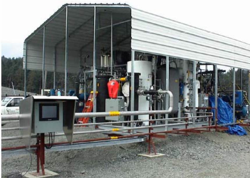
Figure 3-7 Skid-mounted 225-gpd landfill gas liquefaction Hartland Unit, located in Victoria, B.C. developed by CryoFuels Systems, Inc. (source: CryoFuels Systems, undated)
