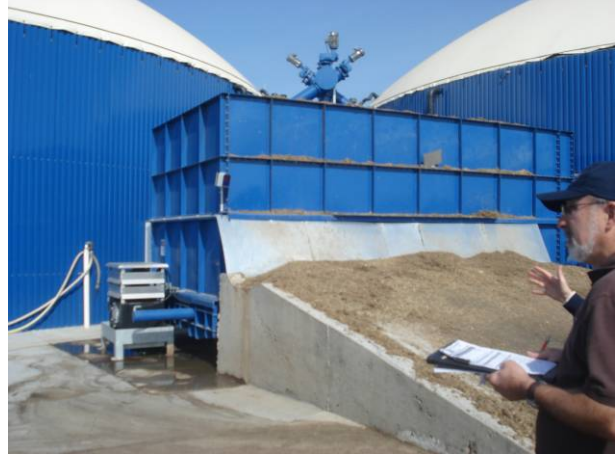
Figure 7.2: Bin for Loading Solids to Digesters.
