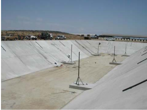
Figure 6.1: Digester Lagoon in Construction.
