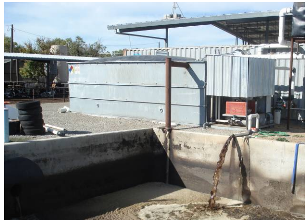
Figure 6.4: H2S Scrubber Behind Receiving Pit.
