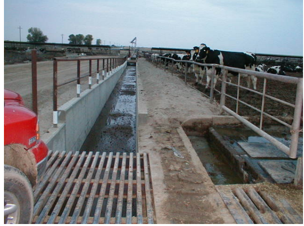
Figure 5.2: Concrete Manure Flush Troughs.
