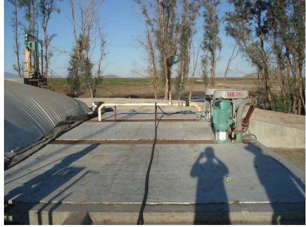
Figure 8.3: Manure Collection Pit at Head of Digester.
