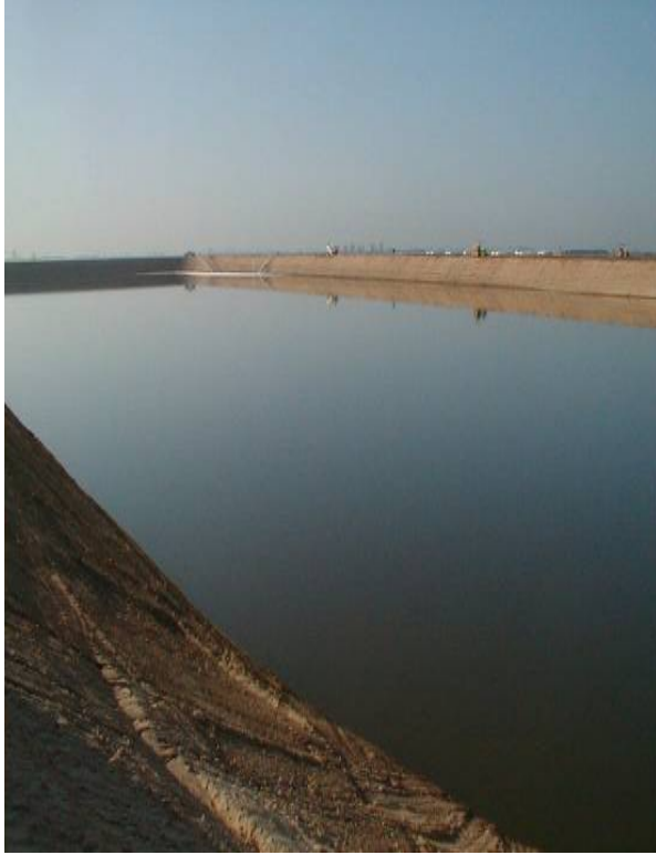
Figure 5.5: Overflow Storage Lagoon.
