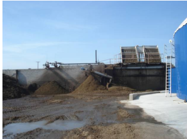
Figure 7.4: Manure Solids Separation.
