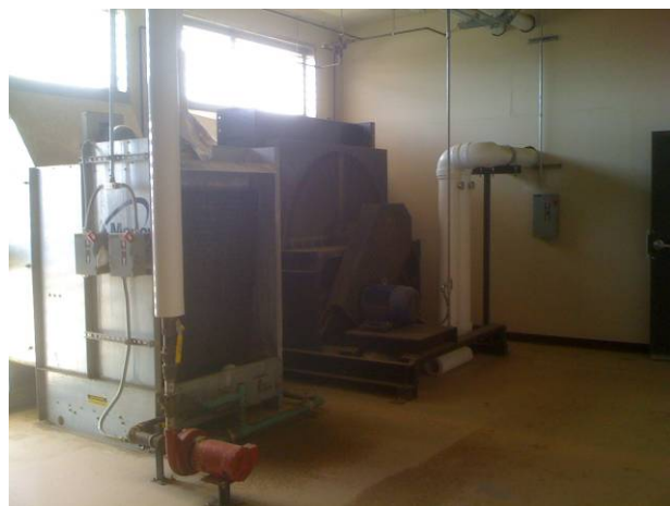
Figure 7.6: Heat Radiators Near Engine Room.
