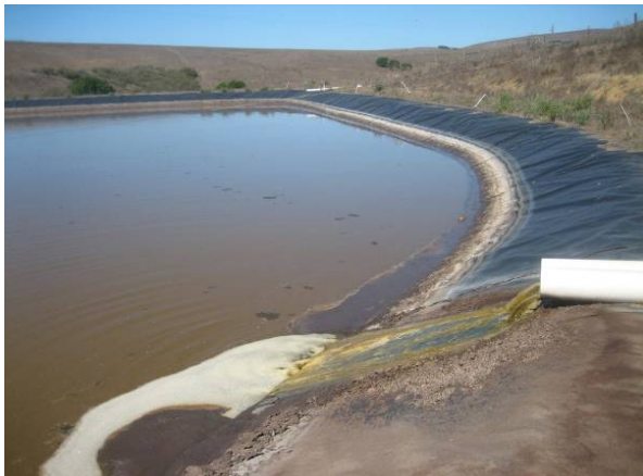
Figure 4.3: Lined Overflow Lagoon.
