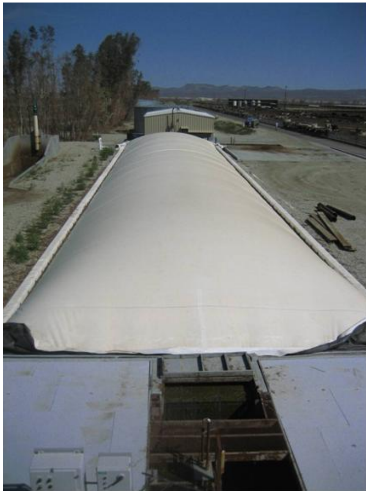
Figure 8.1: Plug Flow Digester System at Meadowbrook Dairy with Generator Building in Background.
