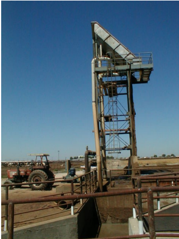
Figure 5.3: Inclined Screen Solids Separator.
