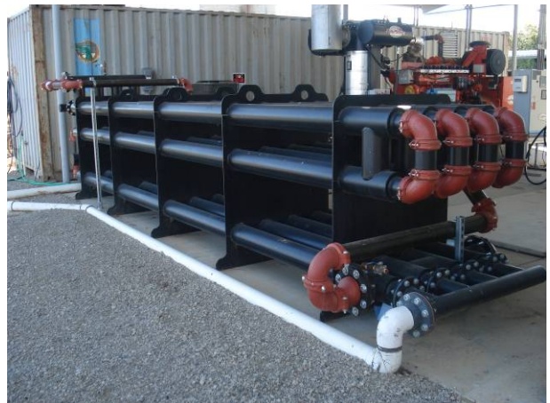
Figure 6.6: Custom Digester Heat Exchanger.
