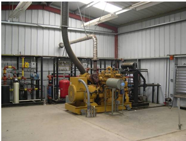
Figure 8.6: Gas Conditioning and Generator.
