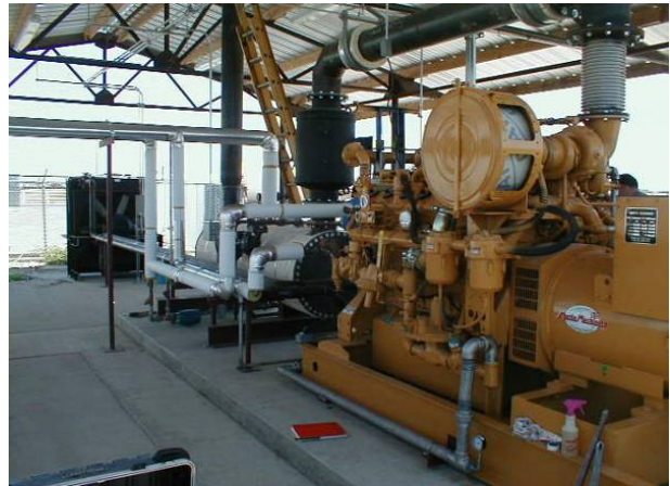
Figure 5.8: 425 KW Engine-Generator with Exhaust Steam Boiler.
