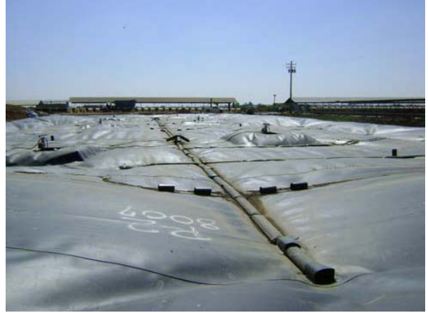
Figure 6.2: Digester with HDPE Cover Installed.
