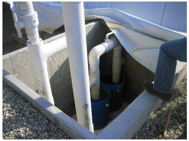
Figure 8.5: Biogas Outlet from Digester.
