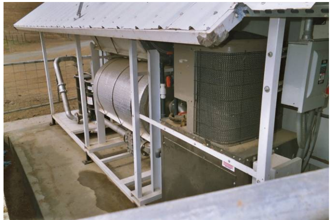
Figure 4.4: Gas Handling Skid.
