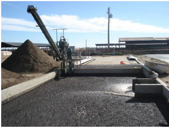
Figure 6.3: Effluent Pit and Solids Separator.
