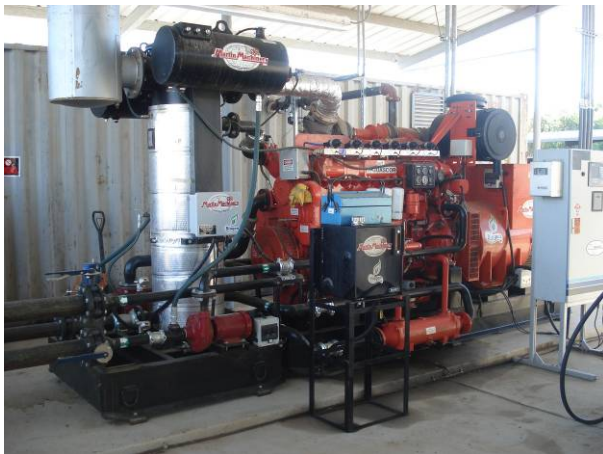
Figure 6.5: 212-KW Engine-Generator System.
