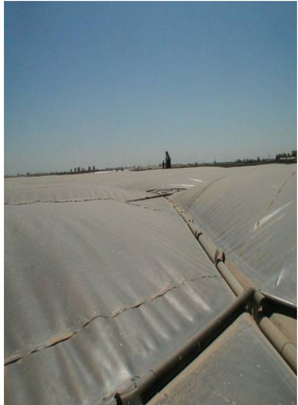
Figure 5.4: Covered Lagoon Digester.
