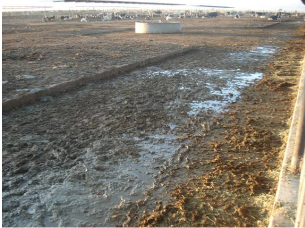
Figure 8.2: Concrete Feed Lanes of Dry Lot Dairy.
