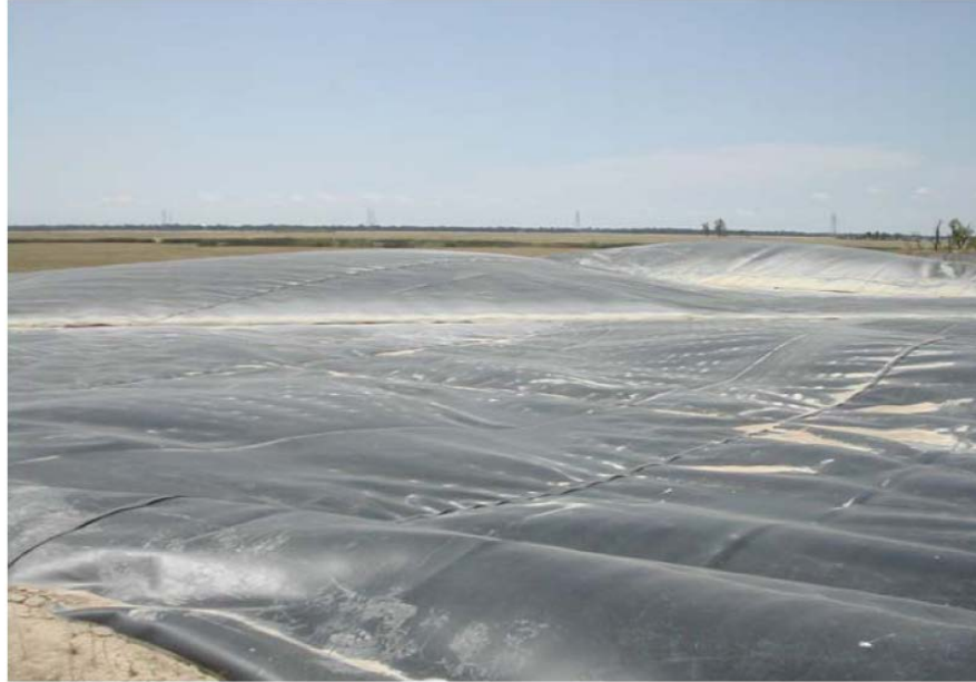
Figure 3.1: Covered Earthen Lagoon Digester at Dairy 1.
