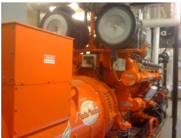
Figure 7.5: 710-KW Engine-Generator System.
