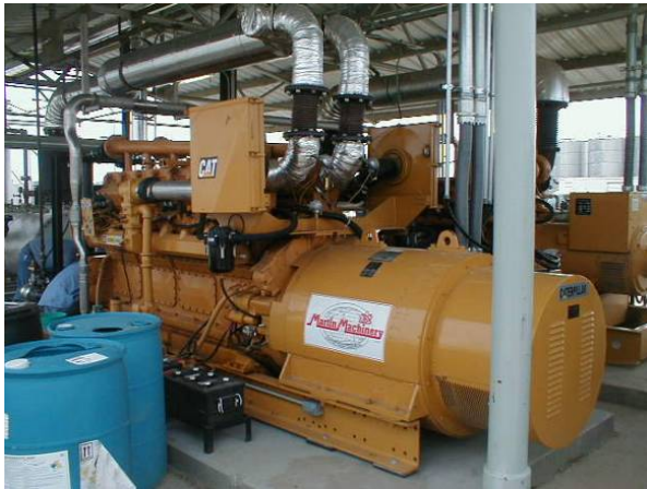
Figure 5.7: 325 KW Engine-Generator.
