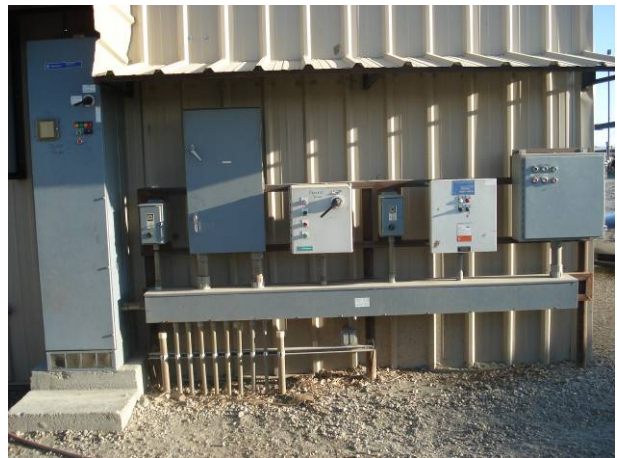
Figure 8.7: Electrical Controls for Digester.
