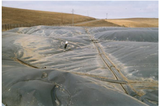
Figure 4.2: Covered Lagoon Digester.
