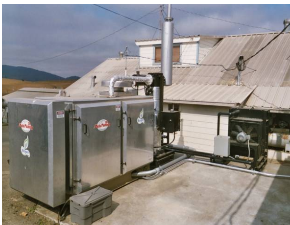
Figure 4.5: 75-KW Engine-Generator System.
