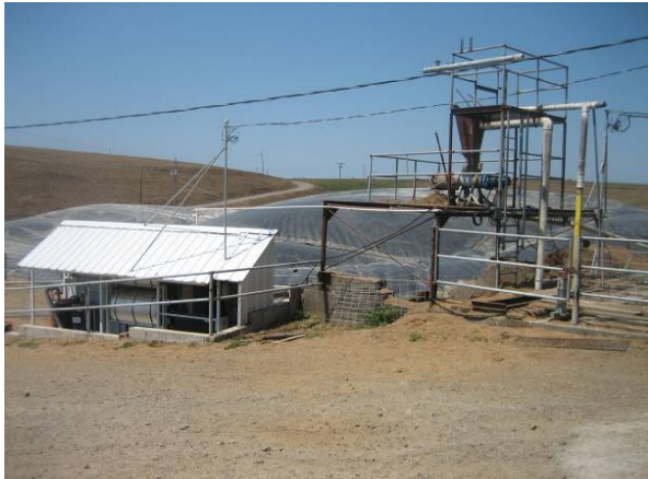
Figure 4.1: Screw Press Solids Separator.
