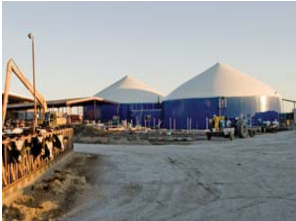
Figure 7.3: Complete Mix Digester Tanks.
