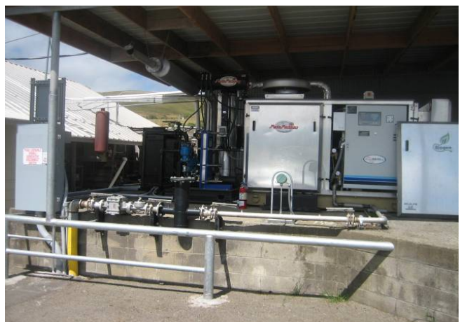
Figure 4.6: Heat Exchanger (Left) Next To Engine.
