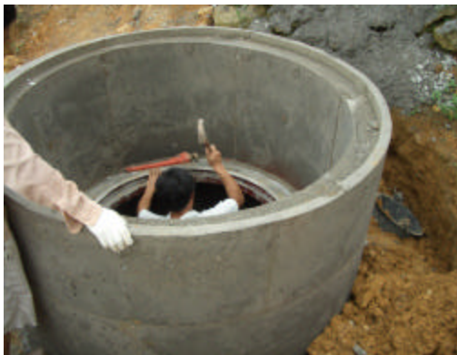
Final Construction of Upper Neck
