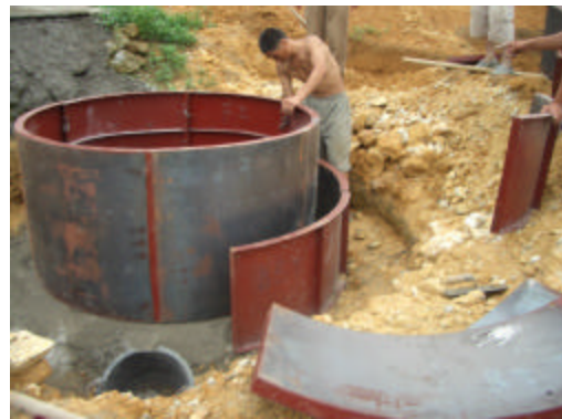
Fitting Upper Mould
