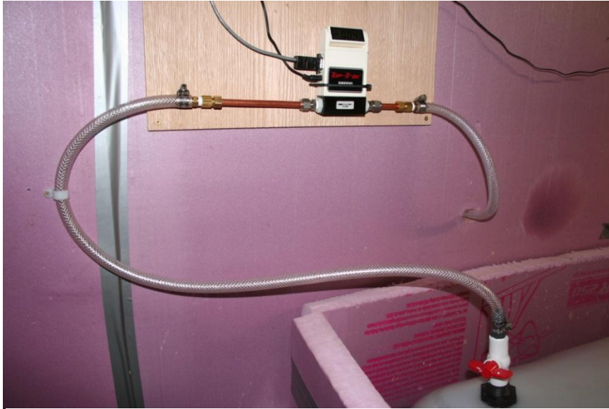
Newly installed gas outlet system. Work was completed retrofitting all tanks on February 25, 2011. The new system only uses standard pipe and gas fittings and the sealant used is Teflon tape. This system is easy to maintain and service in case of future leaks.
