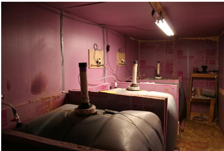
Following the installation of new gas outlets among all of the tanks in the 25°C room each tank began demonstrating the ability to hold pressure. Here each tank is pictured accumulating biogas prior to a venting.
