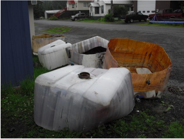
Evacuated tanks had to be cut with a sawz-al in order to be removed and their remaining contents disposed of properly. Photo credit: Clay Koplin.
