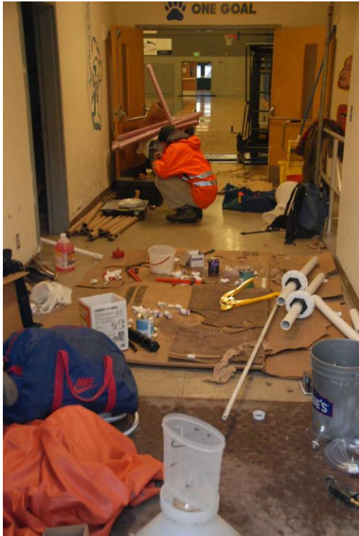
Peter Anthony prepares construction materials.
