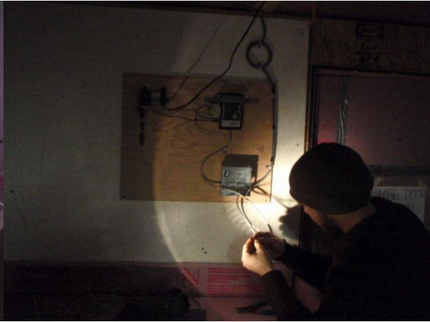
Shaw wires flow meters to a data logger and computer.
