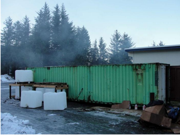
The Conex in first stages of construction behind CHS, with water pressure tanks outside.
