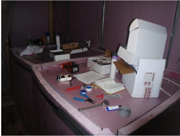
Materials for installing Sierra gas flow meters.
