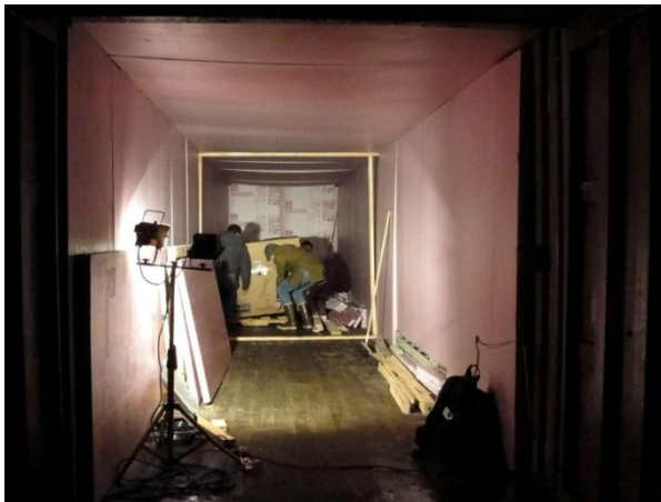
Insulation panels going up inside the Connex, while McFadden and Culhane place the primary slurry tanks.
