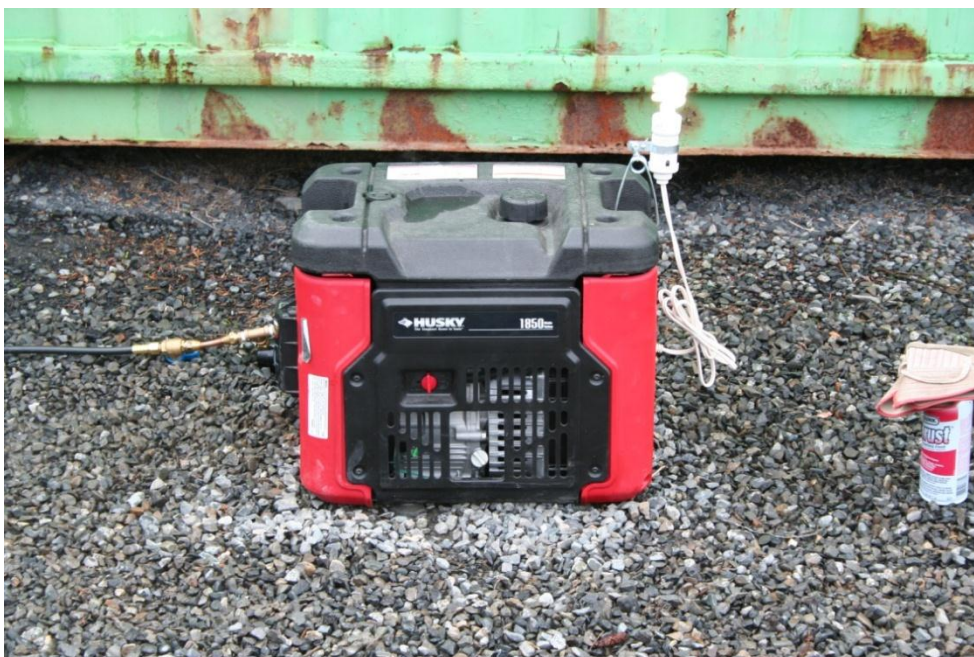
This 1850 Watt Husky generator ran completely on biogas for over an hour before exhausting the biogas storage tank and powering down. Starter fluid was used in order to start the device, but then was sustained entirely on gas collected from inside the Conex (behind). The estimated burn rate for this device is around 1,100 L/hr or 300 gal/hr @ 0.5psi.
