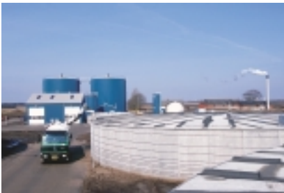
The plant in Studsgaard has positive experience with co-digestion of slurry, organic waste and source separated household waste.
