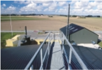
The biogas plant in Hashøj demonstrates combined biogas/natural gas fuelled CHP plant.
