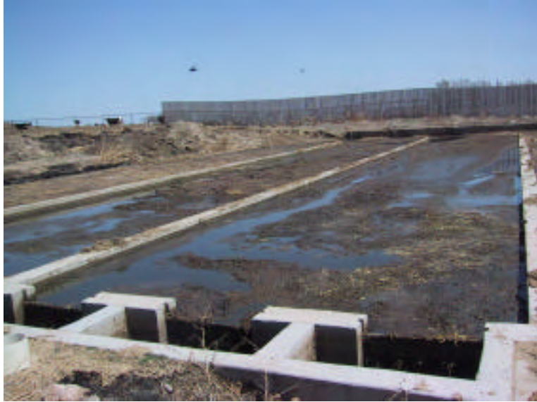
Floating Solids on Top of Gravity Separator
