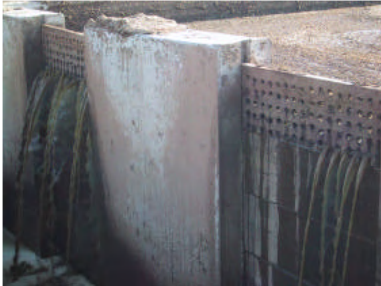
Weeping Wall with Clogged Holes
