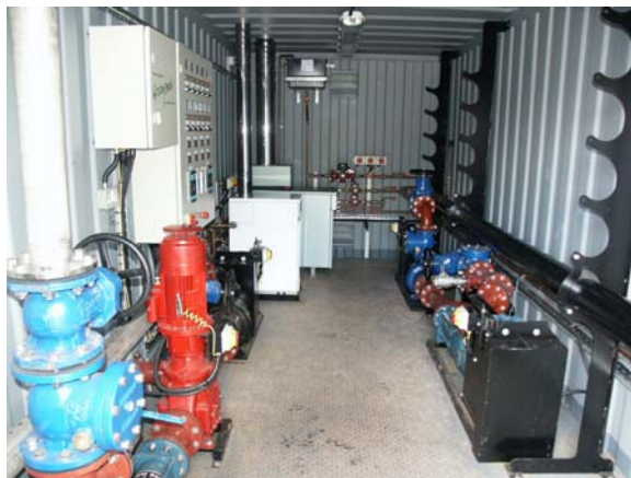
Figure A1.1 Plant Room Container
