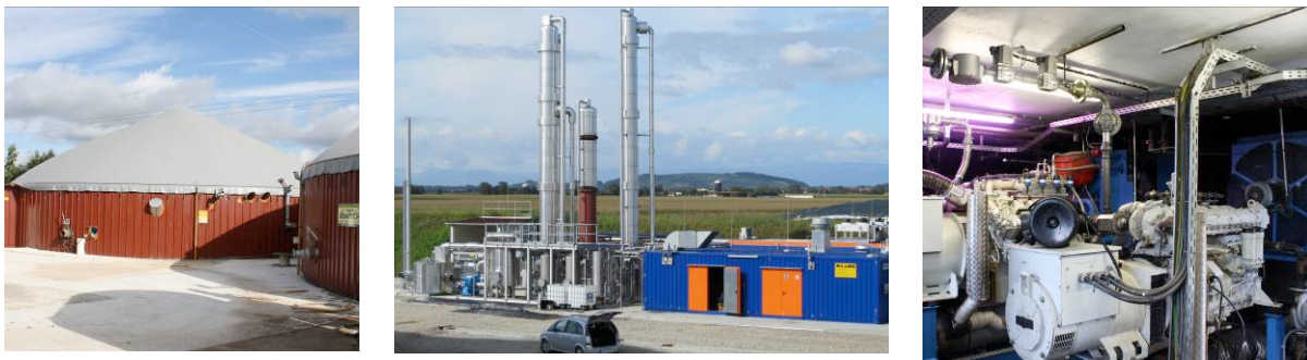
Figure 2. From left to right: (a) An on-farm anaerobic digester, (b) a facility that upgrades biogas to pipeline quality renewable natural gas near Freiburg, Germany, and (c) a combustion engine that converts biogas to electricity.
