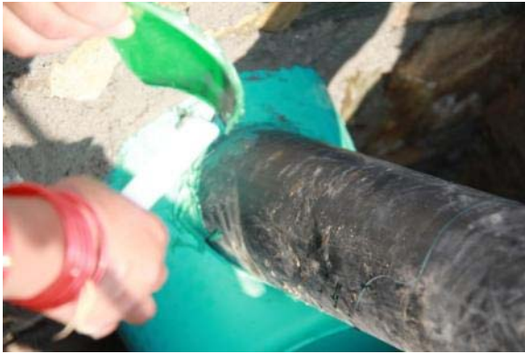
Picture 11: Connect the HDPE-Pipe for inlet/ outlet and fill the gap with liquid concrete (it must be watertight!)
