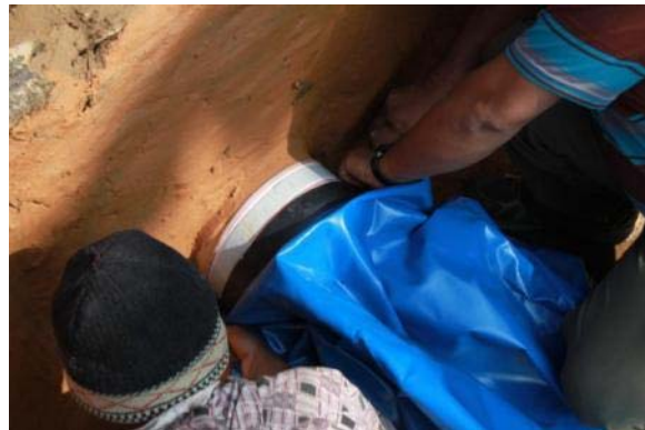
Picture 12: Clean the surface and prepare the Bag Digester. Put the delivered glue on the last ring and attach the Bag.
