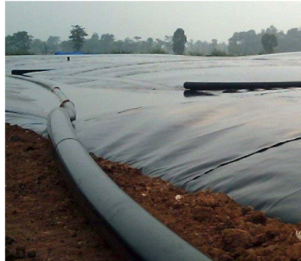
Picture 3: PVC-Bag Digester (Industrial Size) Source: www.alibaba.com
