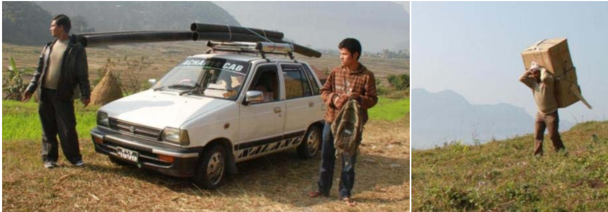
Picture 16: Transport of 2 Bag Digesters in one taxi and carrying of the material to the site (2-3 persons per plant needed).
