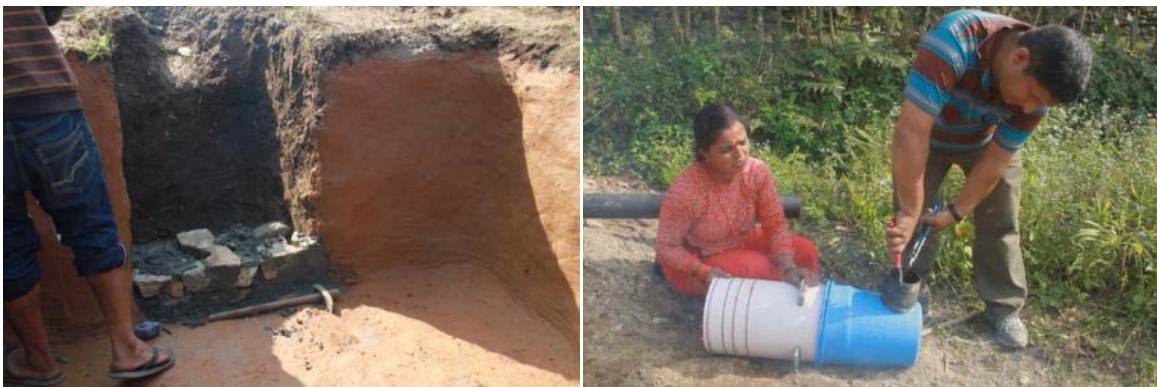
Picture 9: Start the mason work and connect the bucket to the white pipe and make hole with a hot metal pipe
