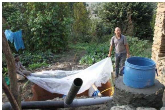
Picture 13: Attach the blue drum as inlet. Construct a bamboo tent for protection.
