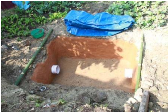
Picture 12: Clean the surface and prepare the Bag Digester. Put the delivered glue on the last ring and attach the Bag.
