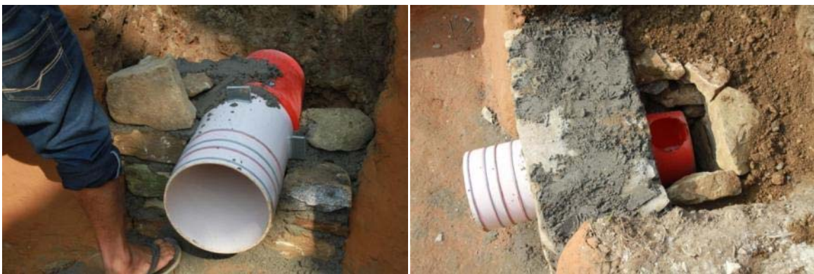
Picture 10: Make the wall (pipe inserted) up to the ground level. Fill the outside with stones & soil up to 4 inches from the red bucket.
