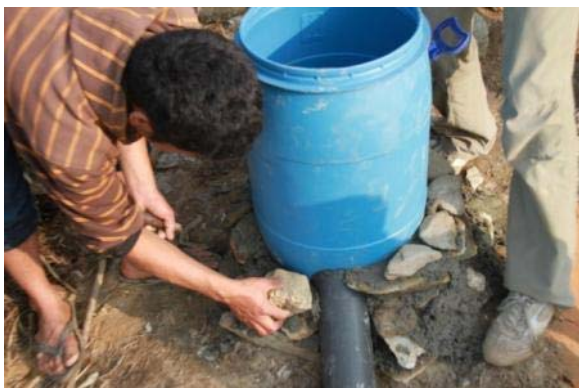
Picture 13: Attach the blue drum as inlet. Construct a bamboo tent for protection.
