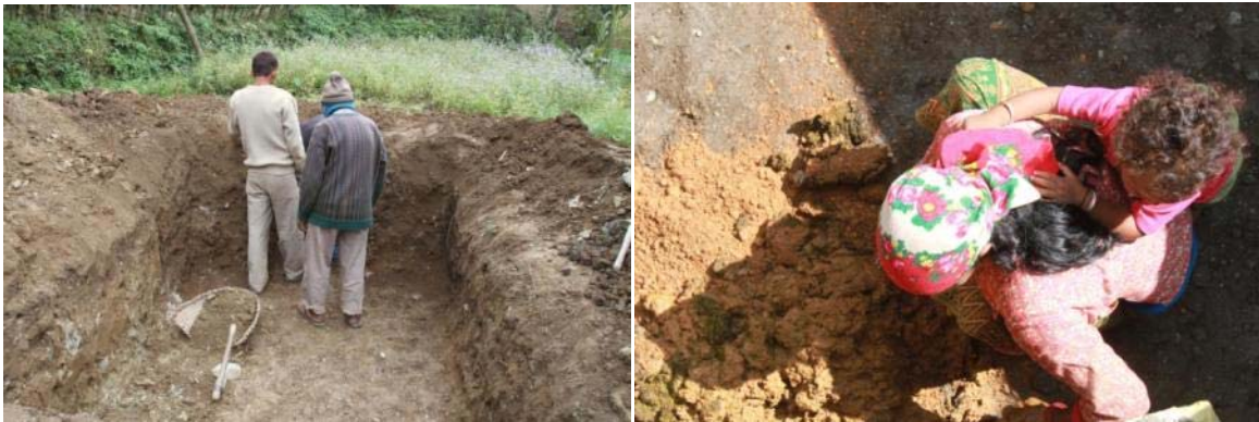
Picture 8: Dig the pit and clean the surface with „Rato mato“
