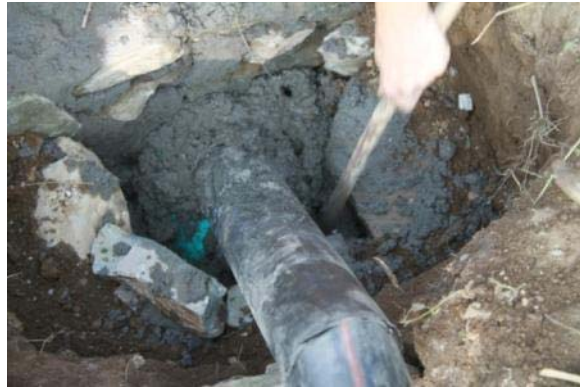
Picture 11: Connect the HDPE-Pipe for inlet/ outlet and fill the gap with liquid concrete (it must be watertight!)
