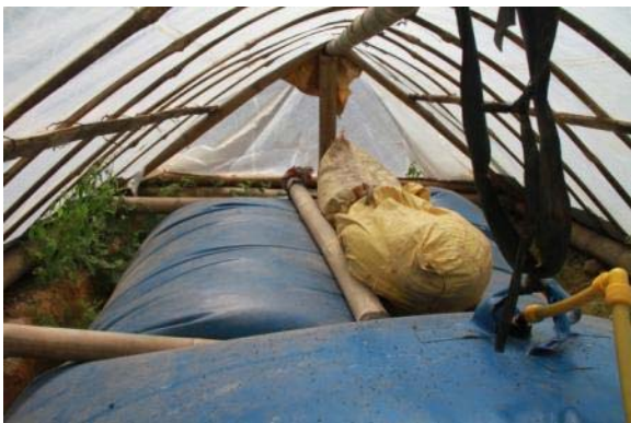
Picture 14: Fill two bags with soil and attach them on a bamboo frame as a weight for the gas pressure.
