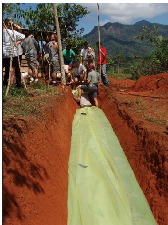
Workshop participants building a micro-scale digester in Costa Rica. Photo by Ian Woofenden.
