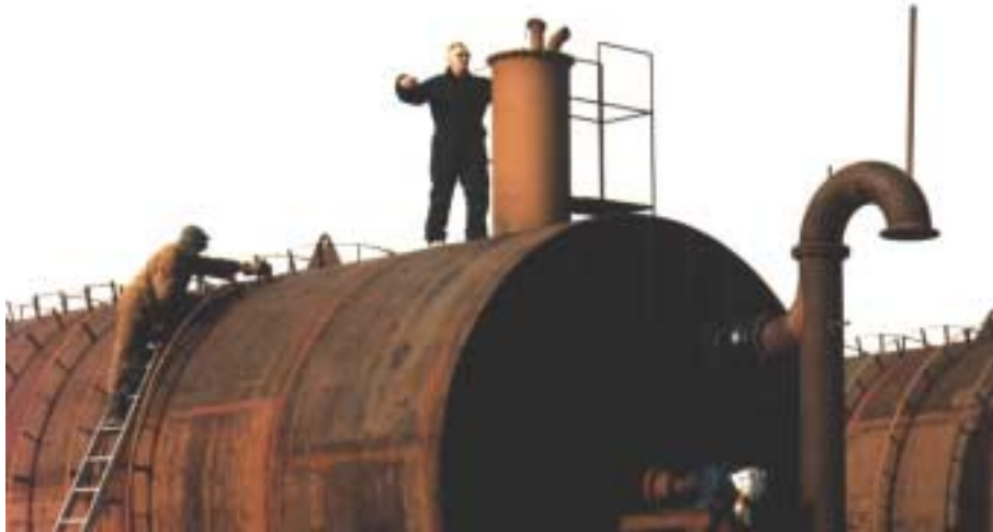
Picture 3-13 The supervisor from the Danish insulation company Scanca takes the last measures before departure to the ICC factory in Mazeikiai, where the prefabrication of the cover plate should take place. At the same time an employee from ICC dismantles the old insulation supports from the digester.
