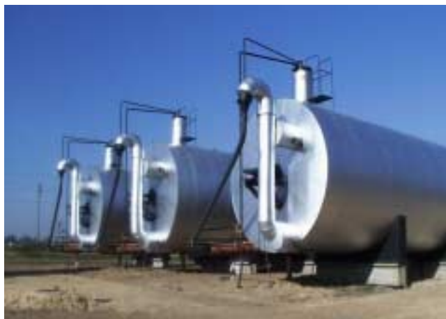
Picture 3-24 The manure and gas outlet of the digesters.
