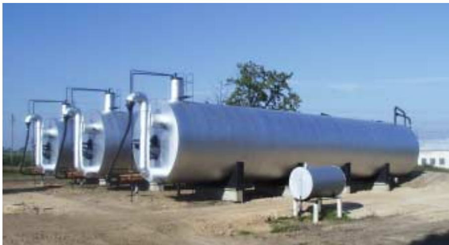
Picture 3-14 In September 1998 it was clear that the efforts transferring technology from the Danish insulation company to ICC was successful. Both the technical quality and the appearance were obviously improved and matched professional western standard.
