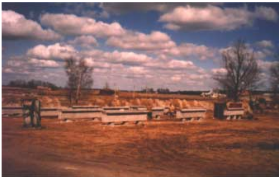
Picture 3-8 The pile foundations were made in January 1997, and the concrete casting part of the foundation was completed as soon as the weather allowed. One digester foot has arrived at the site.
