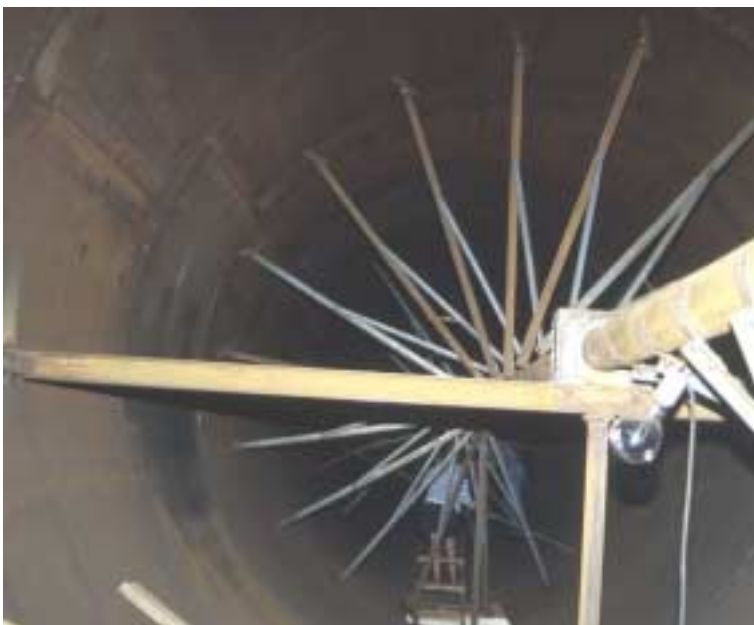
Picture 3-22 A view of the agitator inside a digester. In the foreground is the beam and the oakwood bearing carrying the agitator. On the picture it is still possible to enter through the opening prepared for the sand outlet in the bottom of the digester. Later on, the only way to enter is with a 5 metres ladder through the manhole in the top of the digester. The manhole is seen faintly as a light area in the background of the picture.
