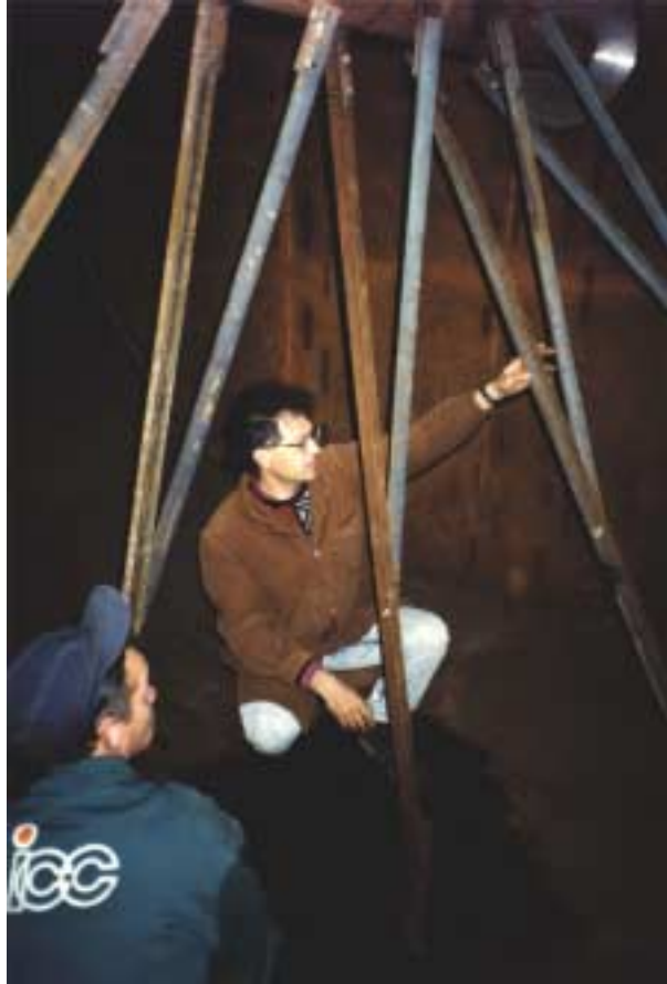
Picture 3-12 There were many details to check during the inspections. On the picture, Mindaugas Stalnionis, Kaunas Energy Office, assists in the inspection of the agitator system in one of the digesters.
