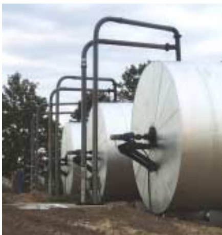
Picture 3-23 Mixer tanks and manure inlet. At the end of the digesters are the motors and gears for the agitators.
