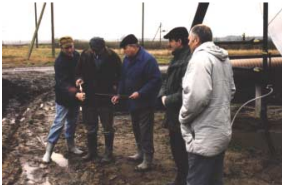
Picture 3-18 Only a few days after the 1 st digester was filled with manure and grafting material, the first biogas flowed in the pipes. On the picture the inflammability of the gas is tested with a hastily constructed torch. It was obvious that it was biogas, but still the quality was too poor to burn.
