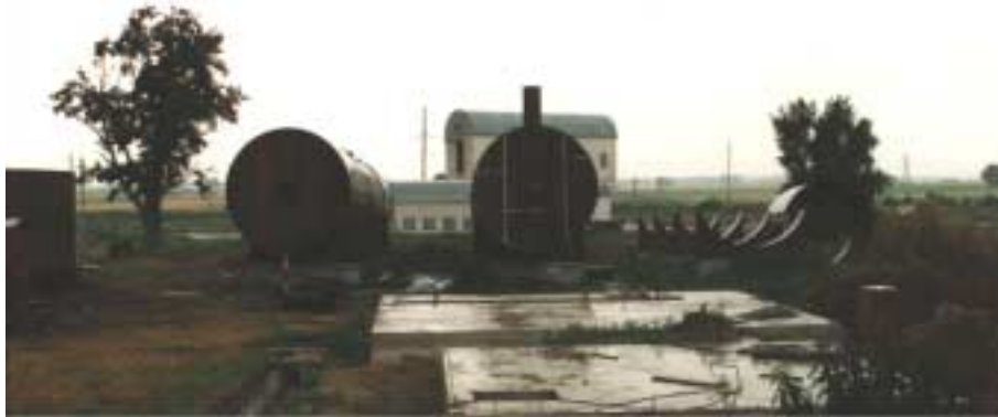
Picture 3-10 The construction site at the inspection in July 1997. Two digesters are mainly constructed, one of them has the agitator system installed. On the right the four digester feet are seen on the foundations, waiting for the main tank for the 3 rd digester. In the foreground of the picture is the foundation for the two technical buildings, motor building and boiler building respectively. In the background are the waste treatment facilities.
