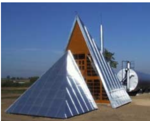
Picture 3-25 The smaller building contains the relatively noisy CHP's. The ground floor of the other building contains boilers and other technical equipment, and the first floor contains laboratory, control system and functions as demonstration area.
