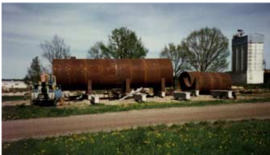
Picture 3-9 The picture was taken in May 1997. The first two of the 4,2 meter diameter and 8 meter long sections of the 1 st digester have been placed on the foundations. The last one is still on the ground where it is welded together from four rings, prefabricated at the ICC factory in Mazeikiai, and welded together at the site.
