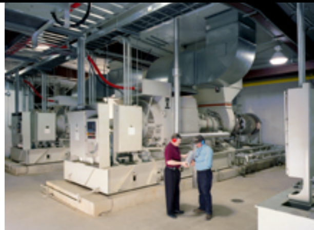
Peaking Power Taurus 60 Turbine Generator Sets, Rural Electric Coop, U.S.A
