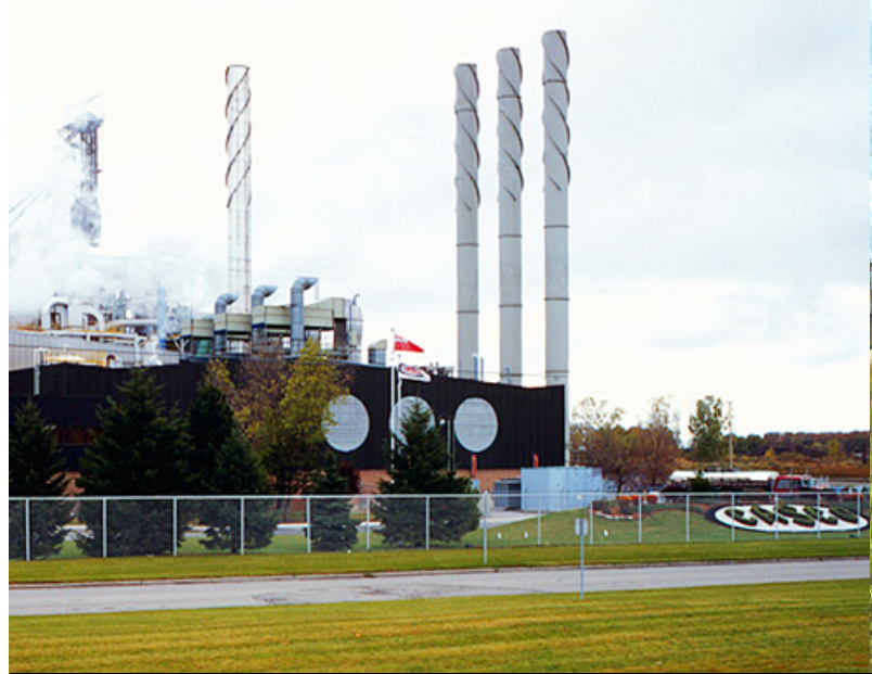
Industrial Cogeneration Taurus 60 Turbine Generator Set, Food Processing, Canada
