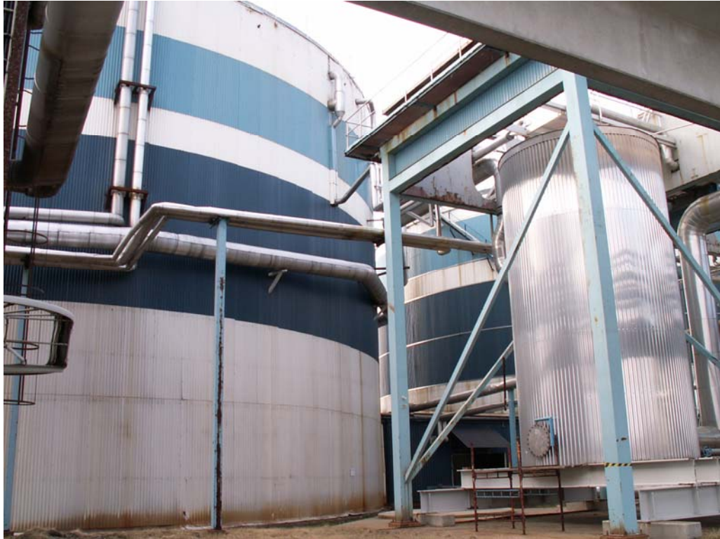
Figure 5.11.1 The biogas plant at Domsjö. The blue and white tanks are anaerobic digesters and the polished steel container is a de-gassing tank.
