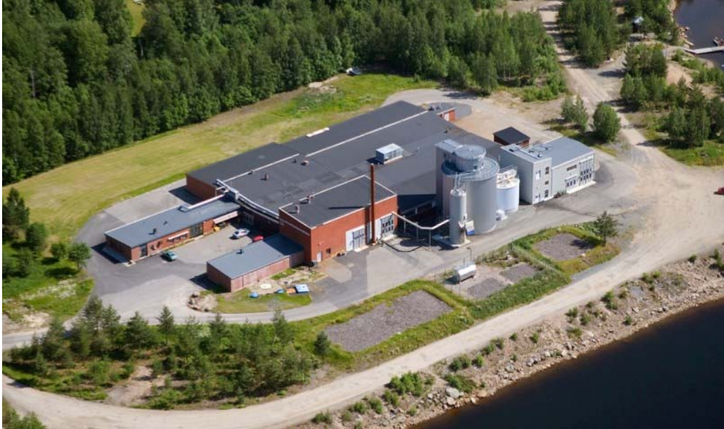
Figure 4.1.1 The biogas plant at Svedjan, Boden
