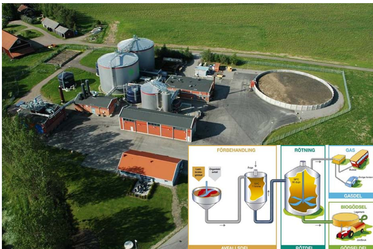
Figure 4.4.2 Aerial photograph of the biogas plant in Linköping, with a schematic diagram of the plant
