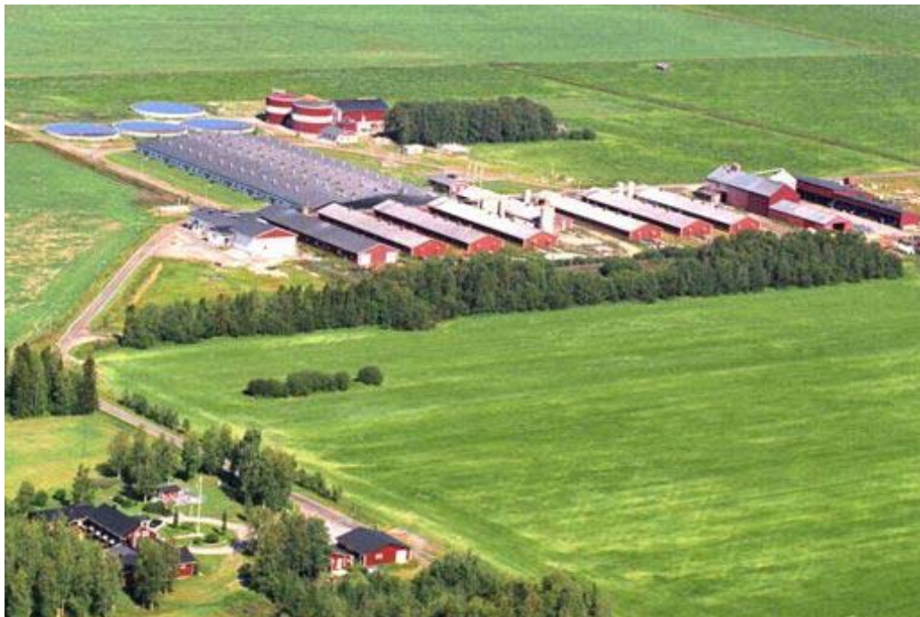
Figure 4.8.1 Photograph of the biogas plant in Alvik
