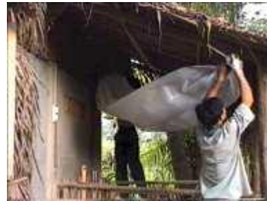
Photo 58. Suspending the reservoir bag in the roof space
