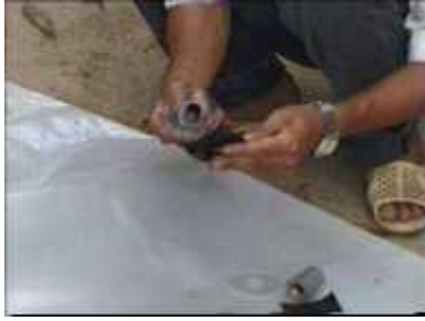
Photo 16. Preparing the materials for the gas outlet
