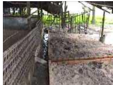
Photo 71. After placing the digester
