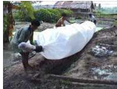
Photo 40. Placing the digester in the trench
