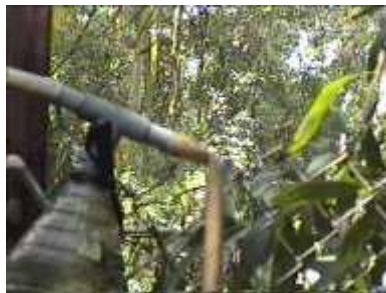
Photo 76. Hose pipe bent down (#4) Cut the damaged hose and join it again
