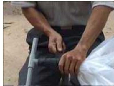
Photo 54. Placing the PVC "T" at the other end of the 3m plastic tube (one of the end of the "T" is joined to the hose coming from the digester and the other to the stove)
