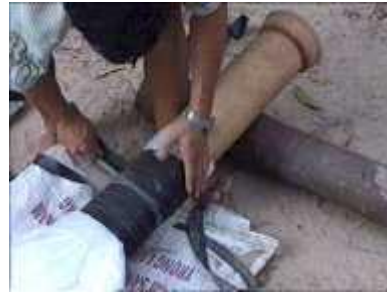
Photo 23. Wrapping the rubber bands around plastic tube where it overlaps the pipe
