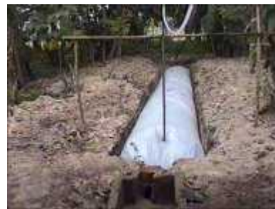
Photo 67. The finished installation
