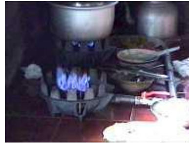
Photo 61. Cooking with biogas
