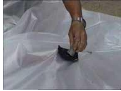
Photo 17. Tightening the gas outlet (without using glue)
