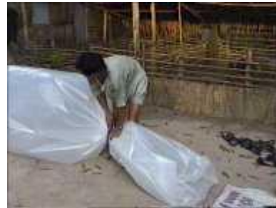
Photo 30. Tying the tube but leaving enough plastic to insert the outlet pipe
