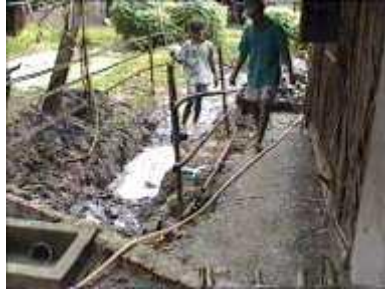
Photo 88. Starting to fix the trench
