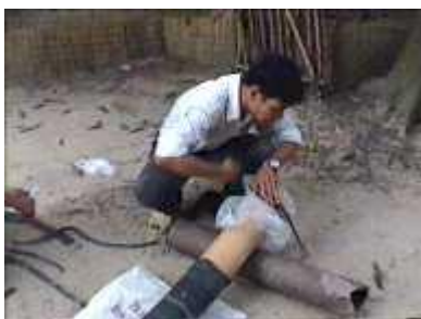
Photo 25. Covering the entrance of the inlet pipe with a plastic bag
