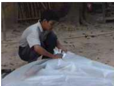
Photo 51. Closing one end of the 3m plastic tube
