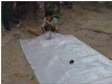
Photo 18. Placing the pipe
