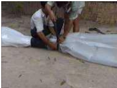
Photo 33. Tying the 3 m length of plastic tube to the exit pipe
