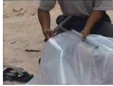
Photo 54. Placing the PVC "T" at the other end of the 3m plastic tube (one of the end of the "T" is joined to the hose coming from the digester and the other to the stove)
