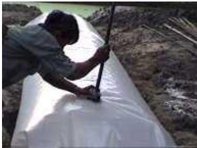
Photo 41. Connecting the PVC pipe to the gas outlet
