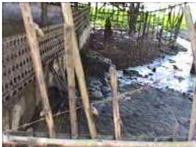
Photo 70. Before placing the biodigester
