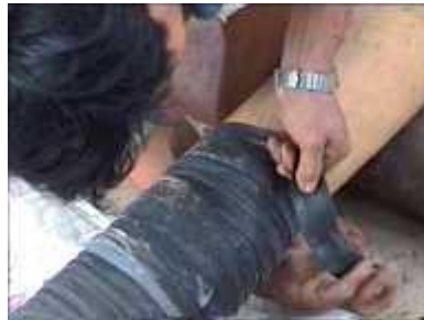
Photo 24. Completing the wrapping of the plastic over the inlet pipe
