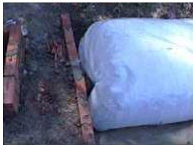
Photo 89. A small wall of brick to avoid the soil entering and rain water entering the biodigester.
