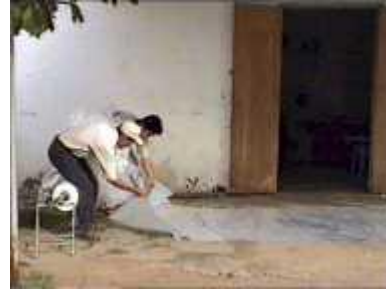
Photo 9. Starting to put one plastic tube inside the other to give added strength
