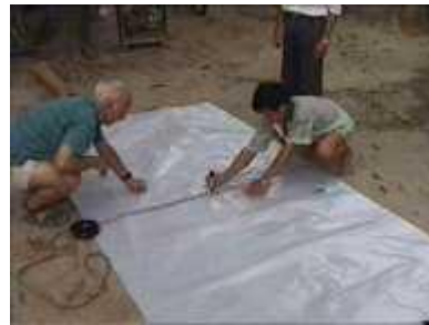
Photo 13. Marking the place to cut the plastic
