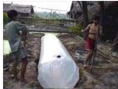
Photo 42. A support is prepared to hold the gas exit line
