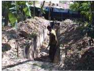
Photo 5. Excavating the soil
