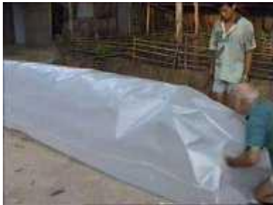
Photo 29. Pumping air until the tube is full
