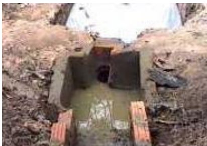
Photo 91. Make a system to capture the sand
