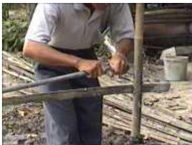
Photo 43. Connecting a plastic hose (or rigid PVC tube) to the PVC gas outlet
