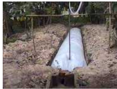
Photo 67. The finished installation
