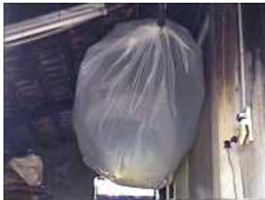
Photo 59. The reservoir bag full of biogas
