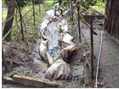
Photo 84. After removing all the content of the digester
