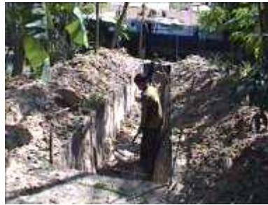
Photo 5. Excavating the soil
