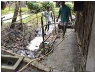
Photo 88. Starting to fix the trench
