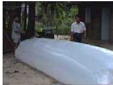
Photo 36. Forcing the air from the 3m tube to the main tube
