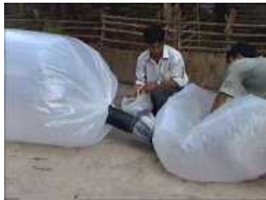
Photo 37. Forcing the air into the main tube until it is full
