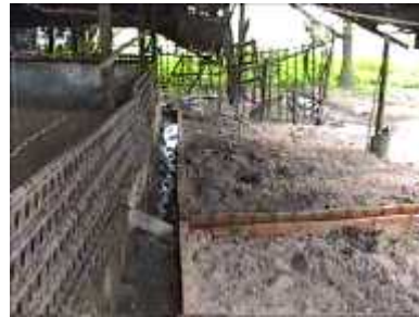
Photo 71. After placing the digester
