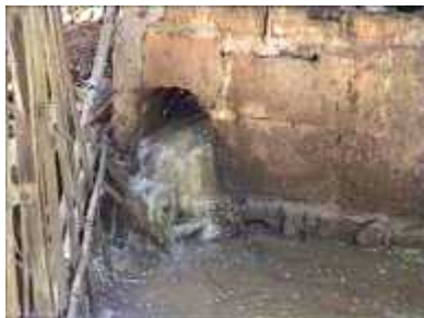
Photo 72. Before placing the biodigester
