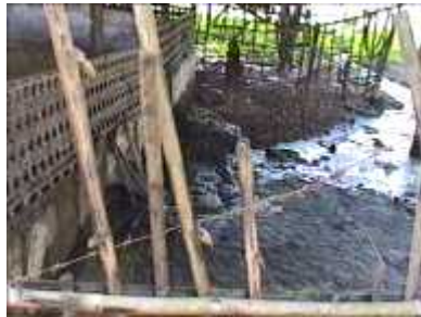
Photo 70. Before placing the biodigester
