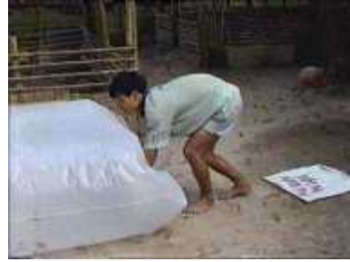
Photo 36. Forcing the air from the 3m tube to the main tube
