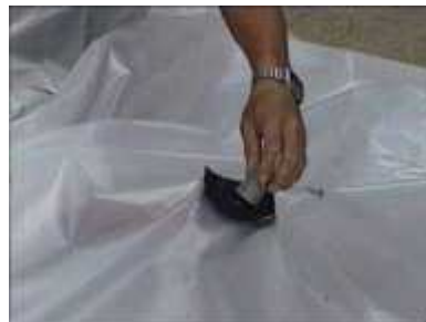
Photo 17. Tightening the gas outlet (without using glue)
