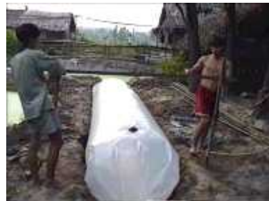
Photo 40. Placing the digester in the trench
