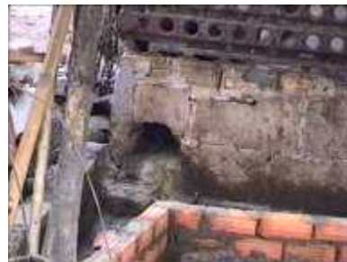
Photo 73. After placing the biodigester
