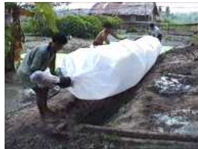
Photo 40. Placing the digester in the trench
