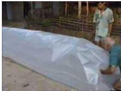
Photo 29. Pumping air until the tube is full
