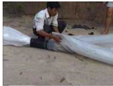
Photo 32. Attaching a plastic tube of 3 m length
