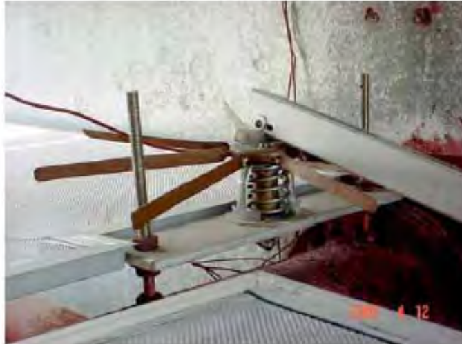
Figure 2.19: Thermostat used in the temperature control mechanism
