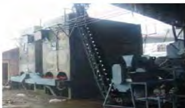
Figure 1. Baguio Composting Facility
