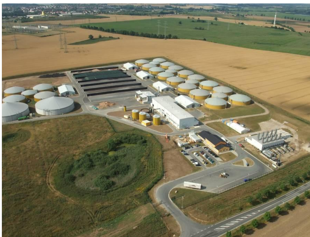
Figure 4. A centralised biogas plant in Güstrow, Mecklenburg-Western Pomerania in Germany. Photo: EnviTec Biogas AG (reprinted with permission).
