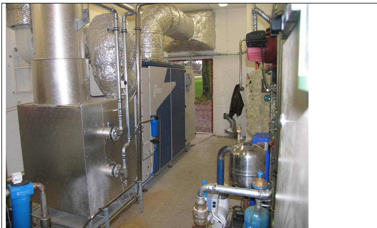
Figure 12. Microturbine installation at Hagavik farm-scale biogas plant, Sweden. Photo:Mats Edström, JTI.
