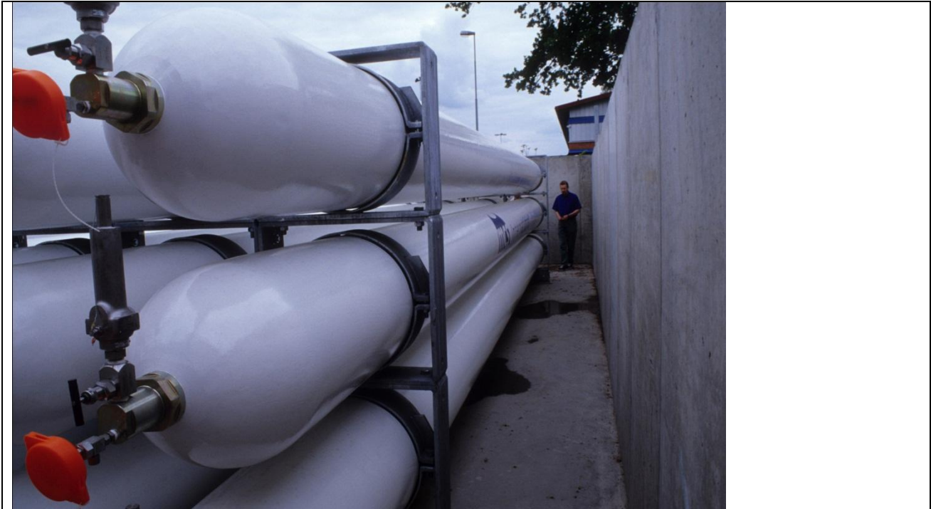
Figure 15. High pressure storage for fast filling of biogas vehicle. Each steel tube has 2000 liters volume and the maximum gas pressure in a tube is 350 bar. Photo: Mats Edström, JTI.
