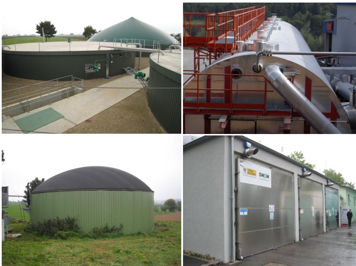
Figure 6. Different digester configurations. Two CSTRs digesting energy crops and a hooded post-digestion tank (top left), A plug-flow digester treating food waste (top right). A farm-scale CSTR treating pig manure and energy crops (bottom left). Garage-type batch digester treating manure from a zoo (bottom right). Photos: Sari Luostarinen & Teija Paavola, MTT.
