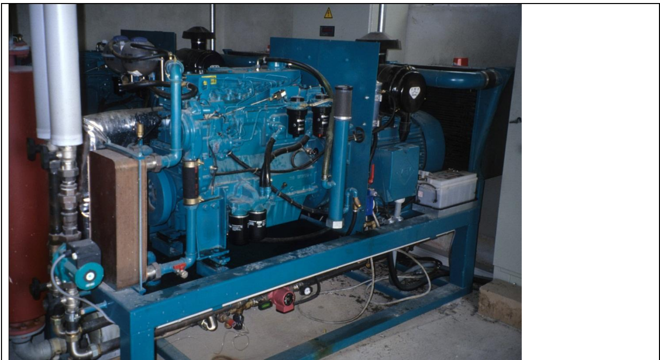
Figure 9. Dual-fuel engine for CHP with biogas. Photo: Mats Edström, JTI.
