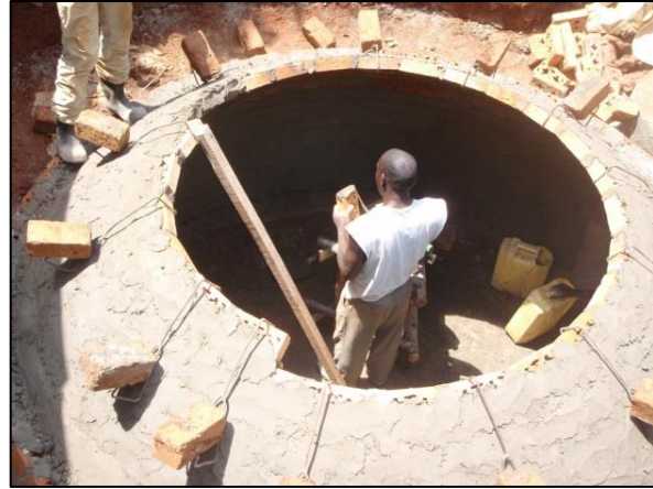
Figure 6: Foundation of a fixed dome (by Green Heat Uganda - GHU)
