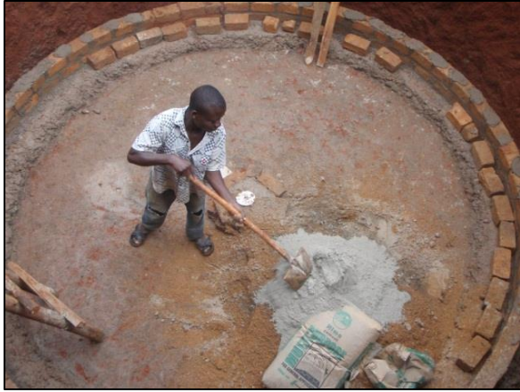
Figure 6: Foundation of a fixed dome (by Green Heat Uganda - GHU)
