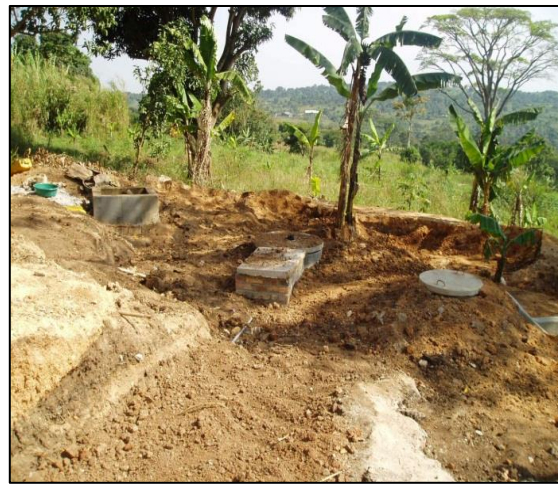
Figure 9: Digester in the ground (by GHU)
