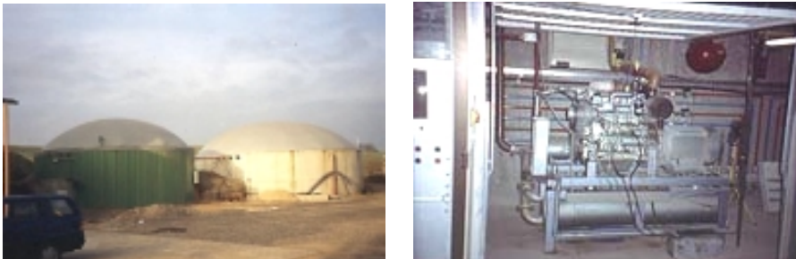
Figure 5. BARZ cofermentation biogas plant and co-generator, Germany.
