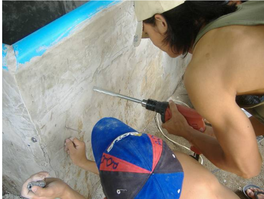
Figure 3.8. Drilling the anchor holes.
