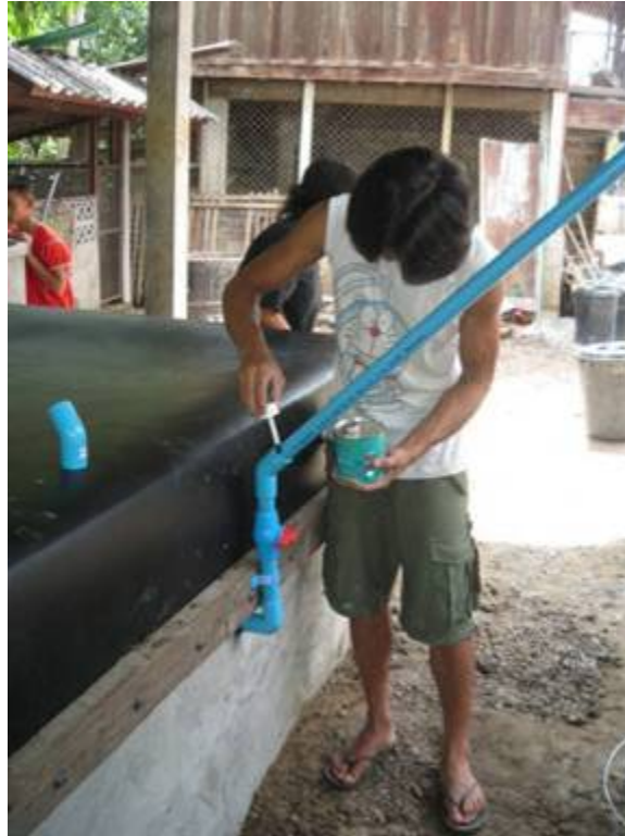
Figure B.10. Gas piping, with valve.
