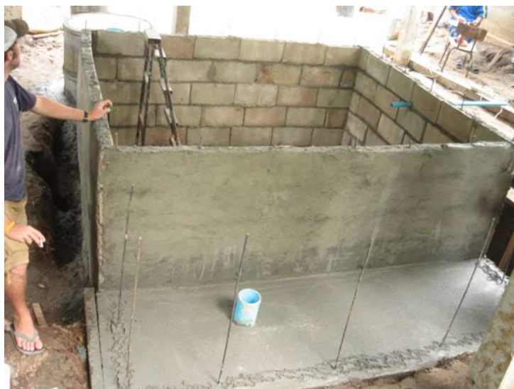
Figure 3.6. The freshly poured outlet tank slab.
