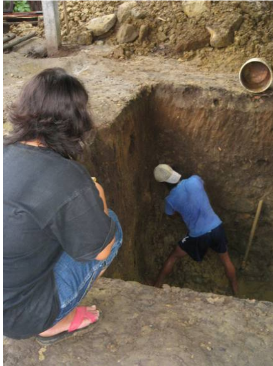
Figure 3.2. The final depth of the hole.
