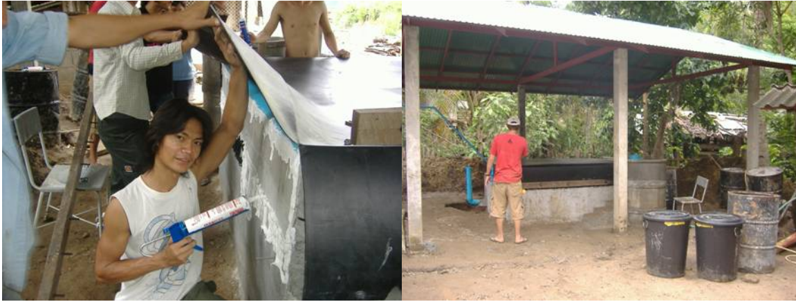
Figure 3.9. Applying the silicone and the completed biodigester.
