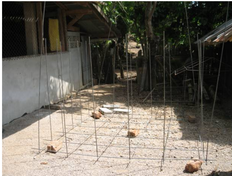
Figure B.1. The rebar structure.
