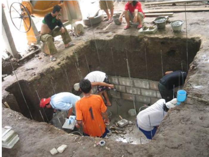
Figure 3.4. Building the CHB walls, with the outlet pipe visible and the hole dug for the inlet pipe on the left.
