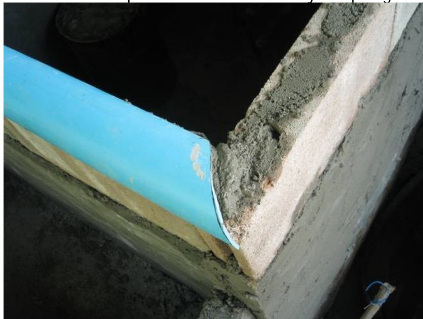
Figure B.5. The PVC used to protect the HDPE from the concrete.
