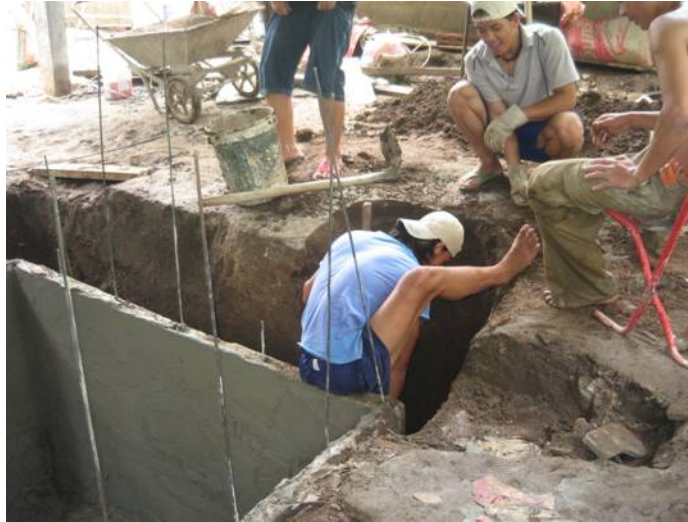
Figure 3.5. Digging the extra hole to alleviate water leaking into the BD.
