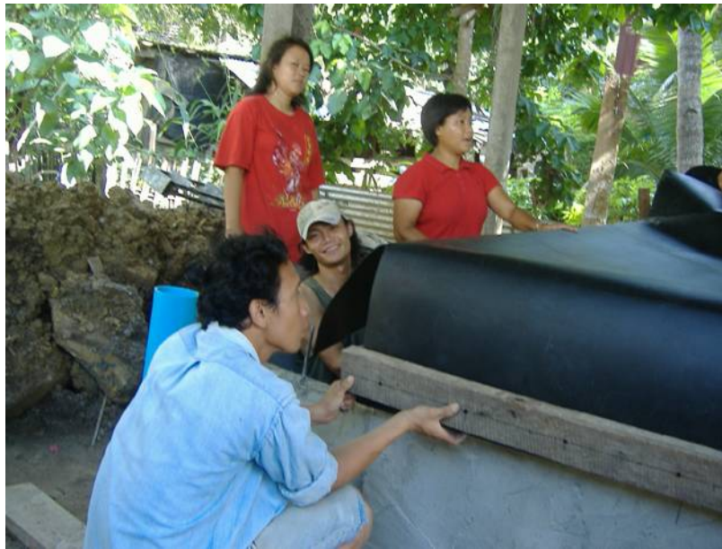
Figure B.6. Positioning the wood to drill through the HDPE.
