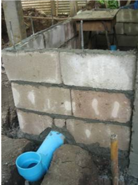
Figure B.4. The drain to the outlet compartment.
