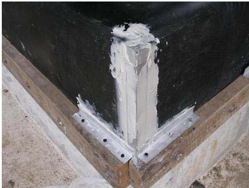
Figure 5.1. Fixed leaks at corners using epoxy glue and aluminum brackets.
