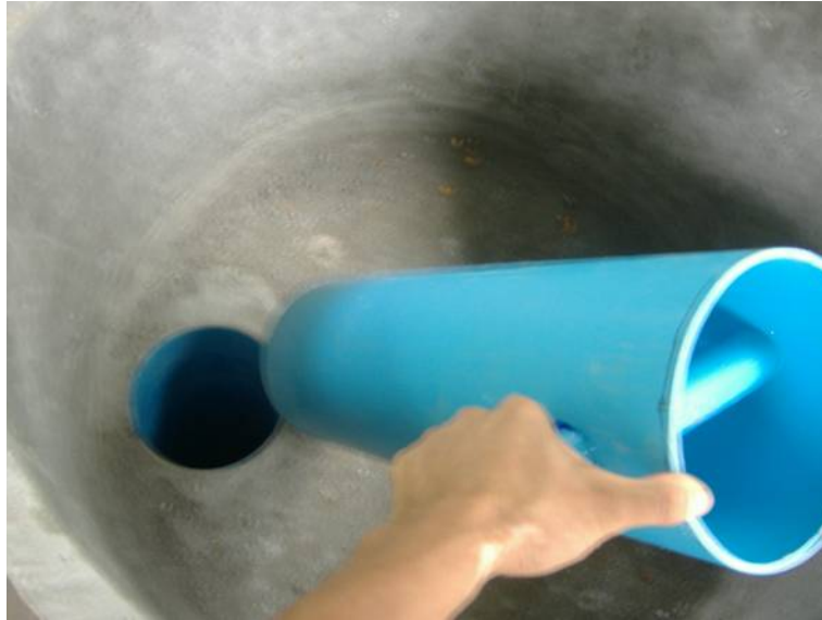
Figure B.9. The length of removable pipe in the mixing tank.
