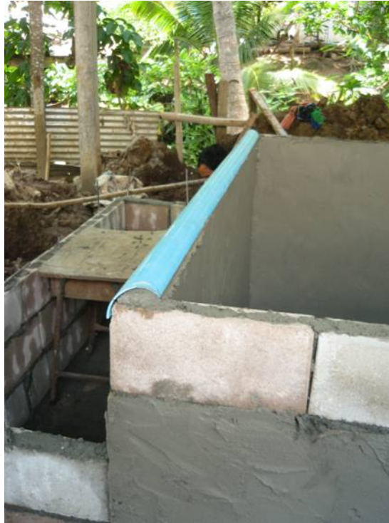
Figure 3.7. The PVC pipe used to protect the HDPE from the concrete.
