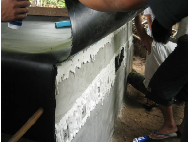
Figure B.7. The silicone to gas seal the BD.
