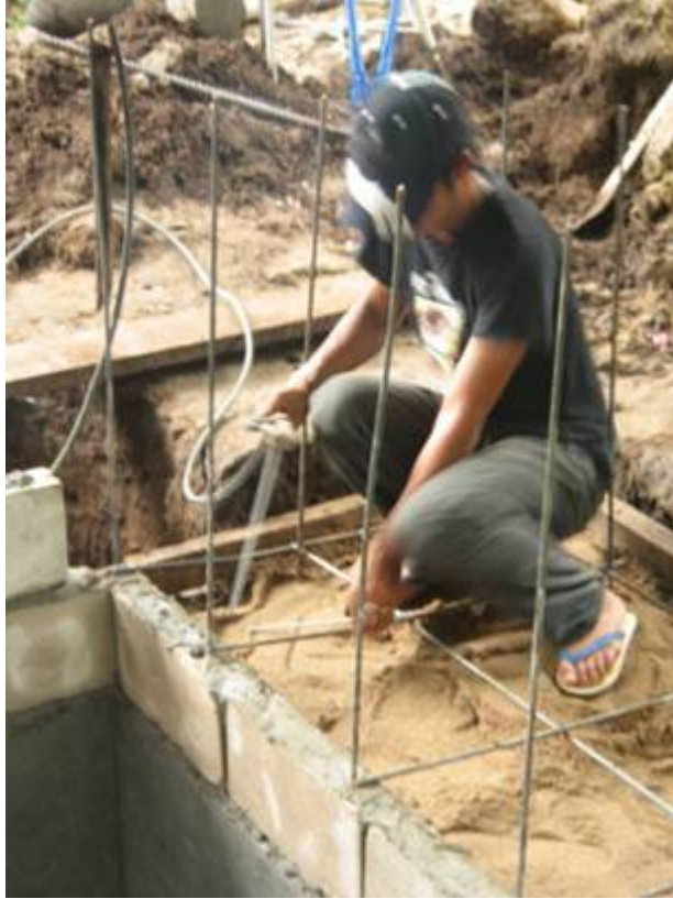
Figure B.3. Placing and welding the rebar for the outlet tank.
