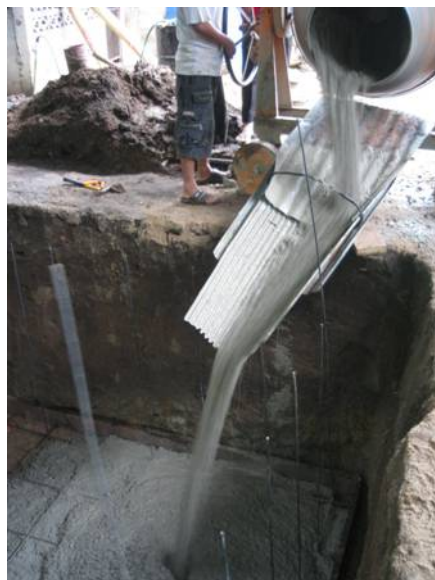
Figure 3.3. Pouring the concrete slab, with the rebar in place
