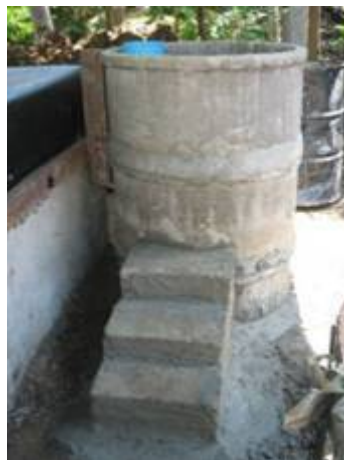
Figure B.8 The mixing tank.
