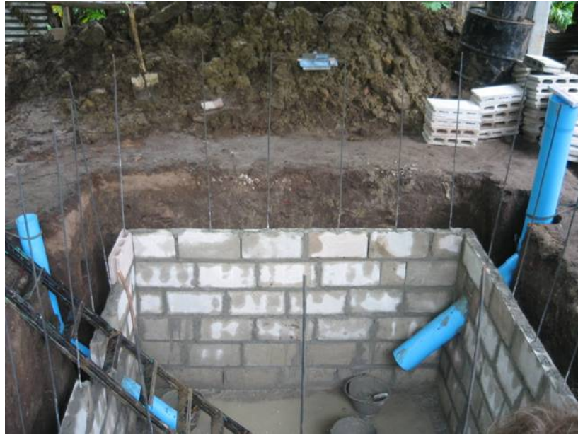
Figure B.2. The inlet and outlet pipes in place, and the pattern of CHB.
