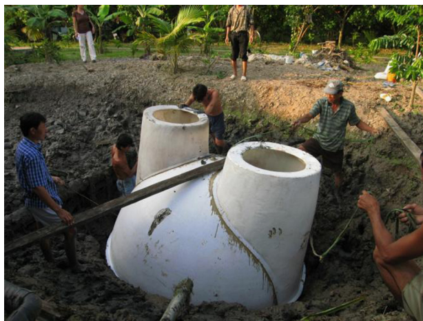
Fig. 6. Installing a household BD at a project site in Vietnam, photo courtesy: Le Thi Thoa.
