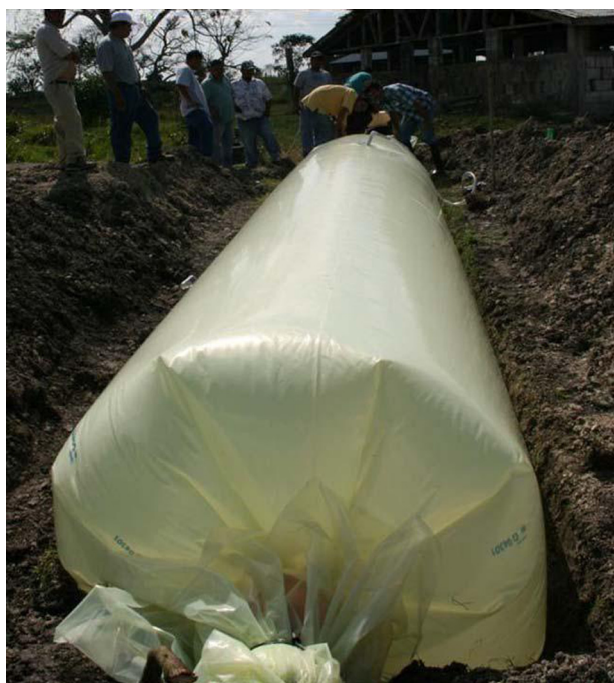
Fig. 2. Installing a low-cost PE tube digester in Belize, photo courtesy: Maximiliano Ortega.
