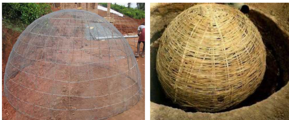
Fig. 9. (Left) Ferro-skeleton-based digester and (right) bamboo skeleton-based digester, photo courtesy: Heinz-Peter Mang.
