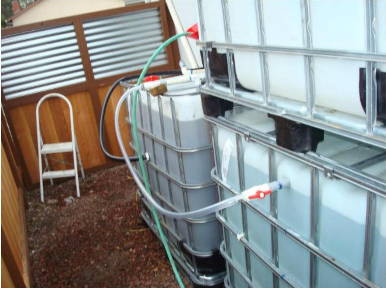
Figure 29. Figure showing how gas is piped from digester to collector
