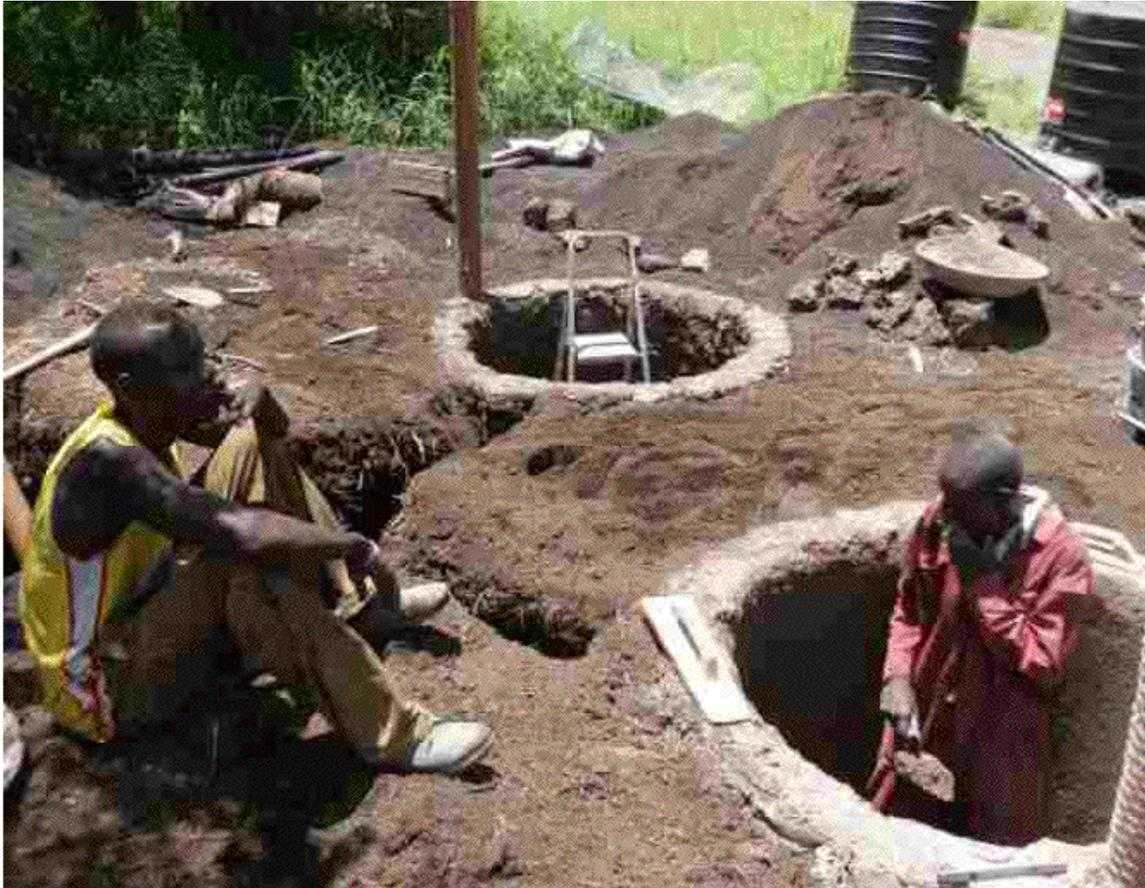
**Figure 35. Digging digestors made from cement in the Ol Donyo Waas conservation area with the Maasai when plastic water tanks were in short supply**
