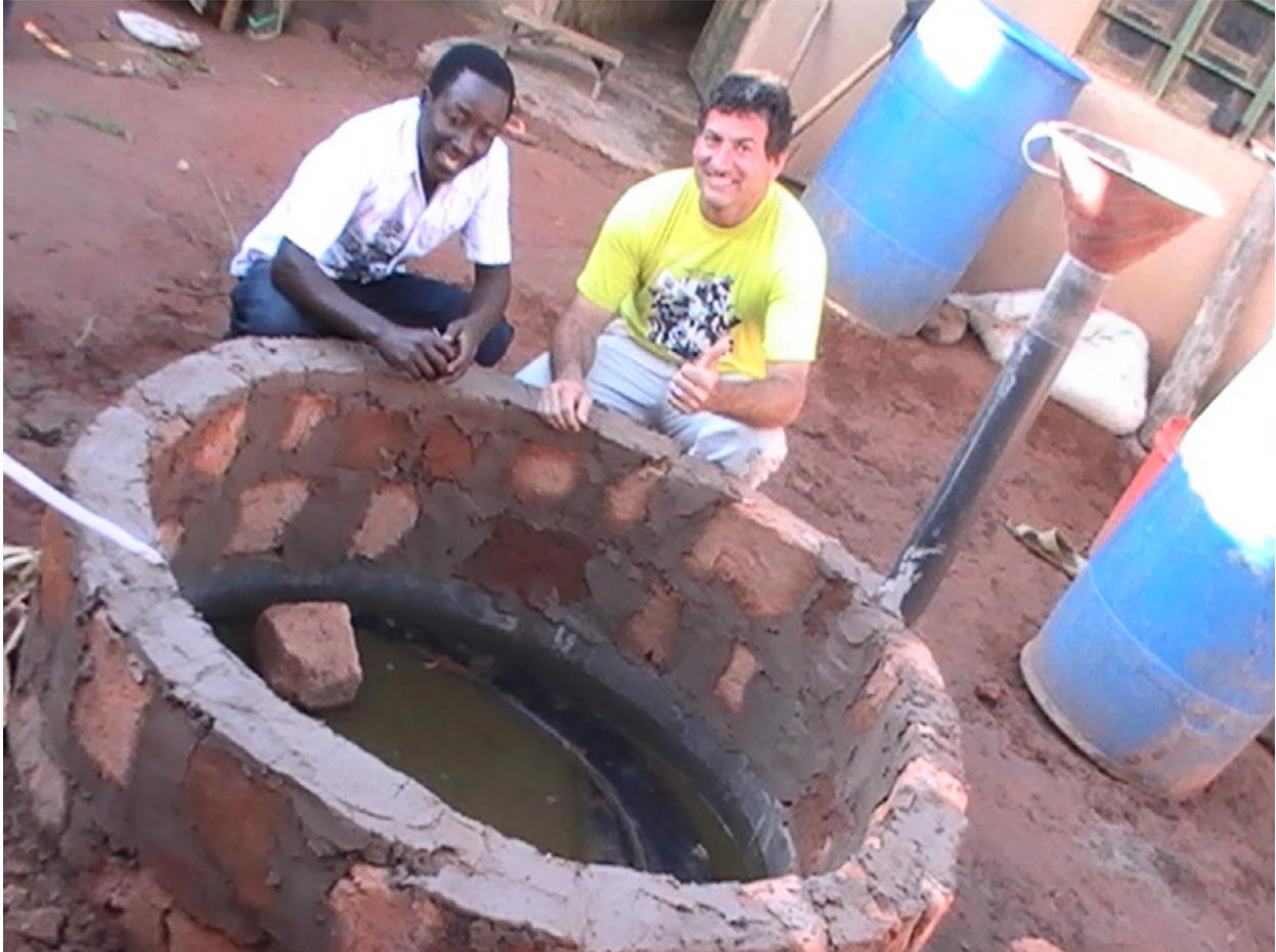
Figure 37. An ARTI style digester with the primary tank made of cement and brick sunken into the ground and a 1000 liter inverted water tank as the gas holder; this solution is advisable when tanks are more expensive or difficult to obtain than cement and brick. The digester need not be submerged – this only adds to the difficulty of making it because of the labor required to dig, but it does allow for eventual connection to an Insinkerator for gravity feeding.
