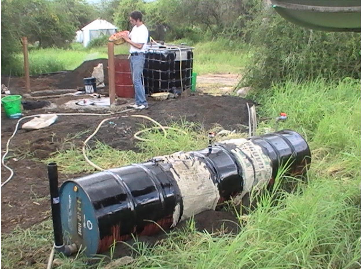
Figure 36. Our Kenyan colleague suggested that we try to make a system out of old oil barrels since plastic water tanks were scarce or expensive. This was similar to an idea the FAO had promoted in Africa in the 1980s. The problem is that it is very difficult to keep micropores from opening up at the weld joints. We had to cover the welds with inner tubes and pitch and still found tiny leaks appearing.
