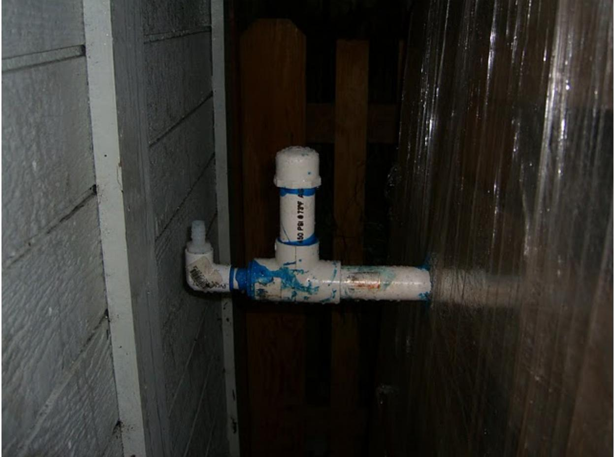
Figure 34. The heat exchanger plumbing
