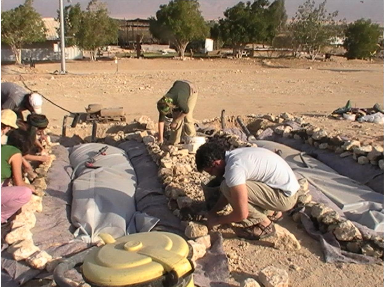
Figure 47. "Salchicha" flexible bag digestors being built at the Arava Institute of the Environment
