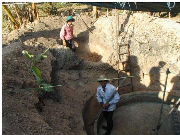
Fig. 6.5.1. Fermentation reactor under construction.
