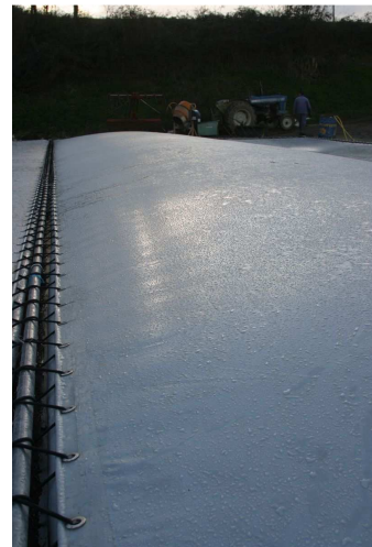
Plastic cover inflated by biogas
