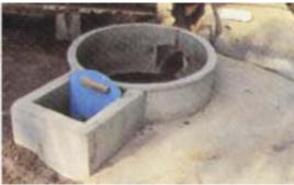
☐ Clean mixing chamber and gate at every addition of the excrement in the digester chamber.
