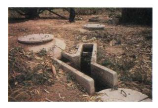
Leave gate opened for a while and after one smells the gas or the overflow slurry is very liquid then close the gate.
