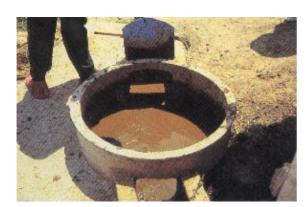
☐ Mix or stir the mixture in the inlet pit until it becomes liquid, then open the gate of the mixing chamber to let the mixture flow into the digester chamber.
