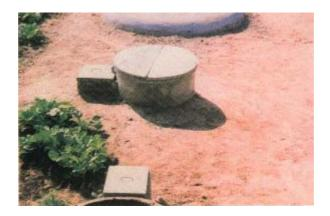
☐ The inlet should be covered to prevent domestic animals from drinking this water and also prevent the water from evaporating quickly.
