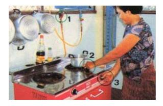
☐ When stove is being used, open valve in the kitchen first and set fire prepared at burner then turn on the switch of stove last.
