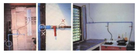
☐ Gas pipe should be installed against the wall or post and secure tightly. The pipe will be broken easily if installed independently or loosely.
