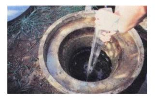
☐ The cover of the inlet pipe should be opened for maintenance once a year. The crust or scum formed by manure should be removed if possible.
