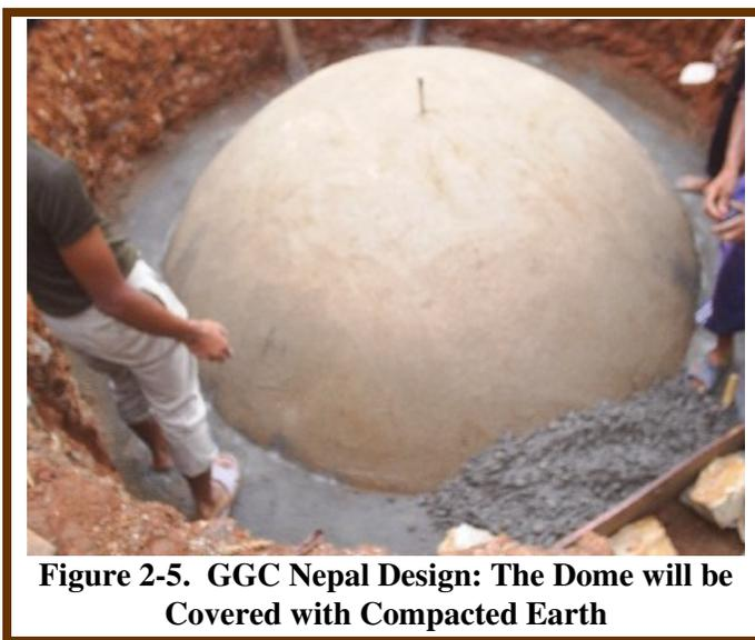
**Figure 2-5. GGC Nepal Design: The Dome will be Covered with Compacted Earth**
