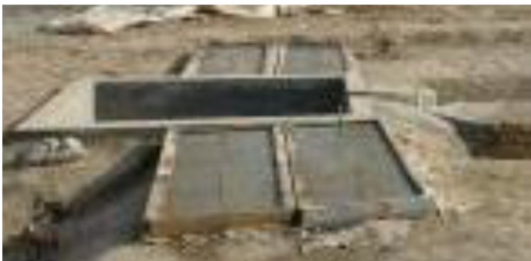
Figure 6.7.1: Outlet chamber slabs in casts.
