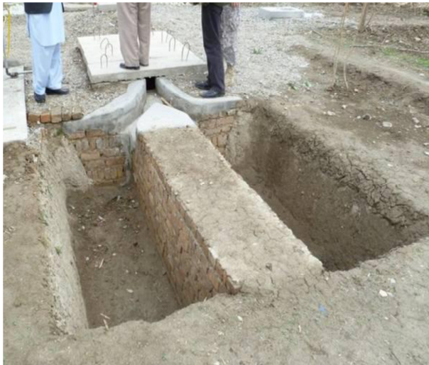
Figure 6.10.1: Compost pits with brick walls for stability
