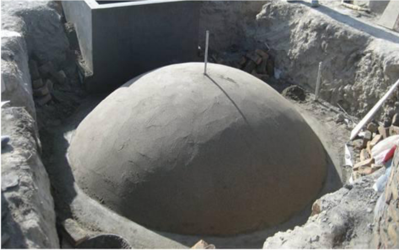
Figure 6.6.2: Earth mould with sand layer before placing cast
