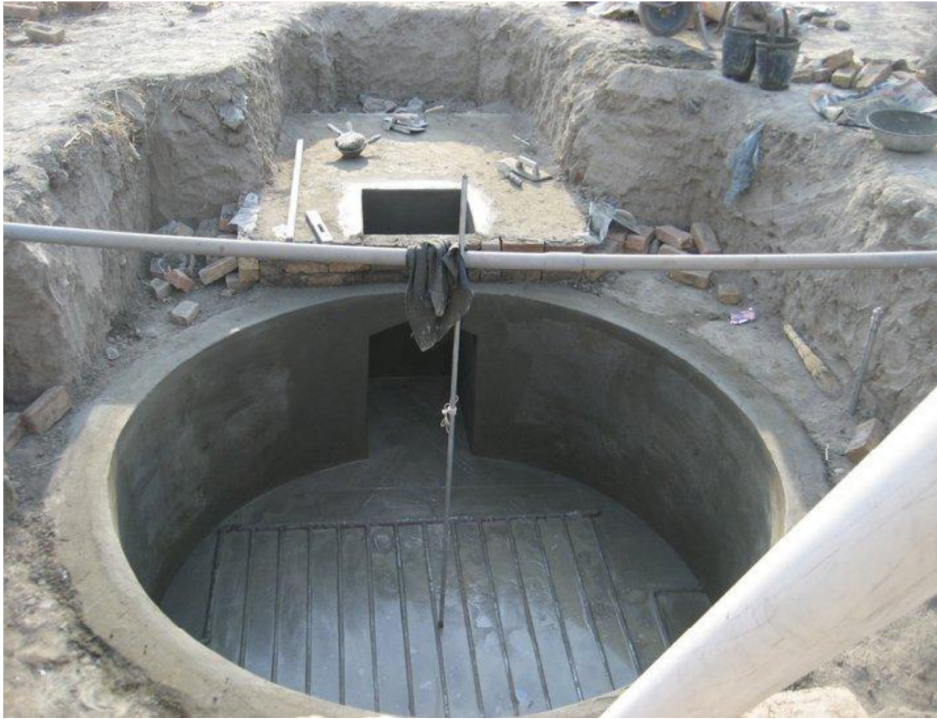
Figure 6.5.3: View of Manhole in Main Digester
