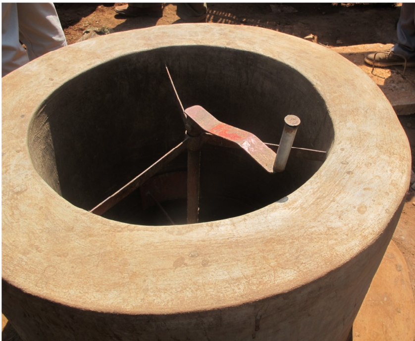
Figure 6.8.3: Complete Inlet Tank with mixer device
