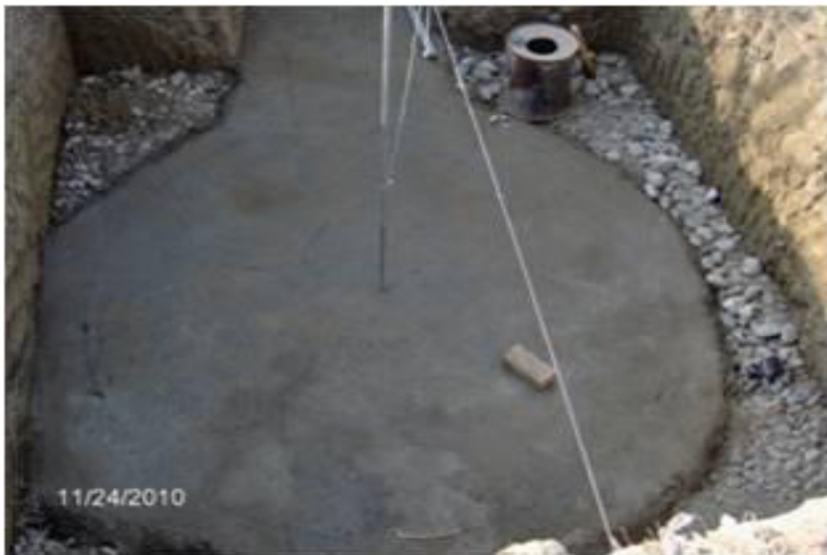
Figure 6.5.2: Concrete Foundation for Digester, Center Guide Pipe and Horizontal Cord.
