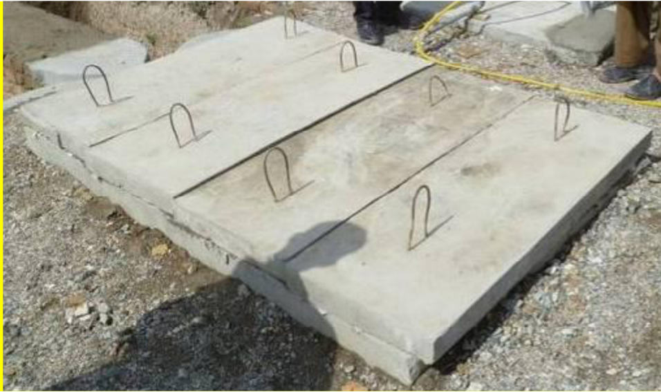
Figure 6.7.3: Slabs in place on outlet chamber
