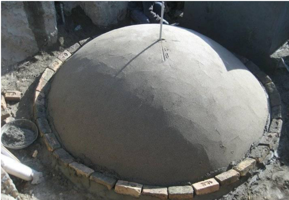
Figure 6.6.3: Earth mould with sand layer before placing dome
