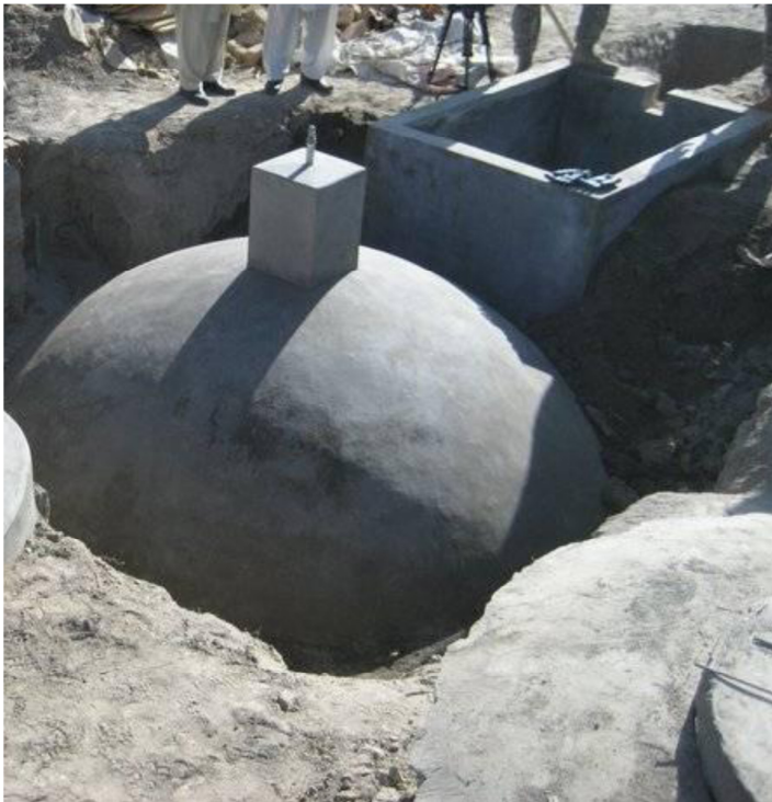
Figure 6.6.4: Completed dome with turret.
