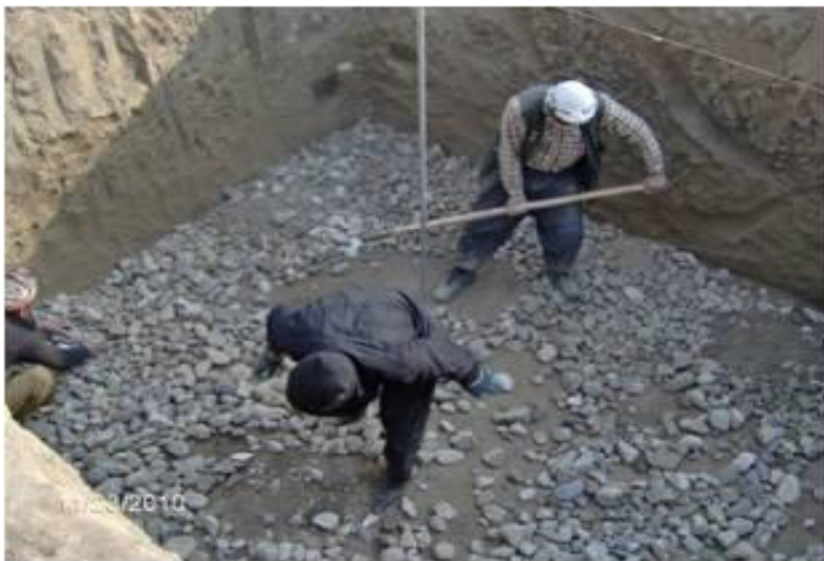
Figure 6.5.1: Cobblestones and Gravel placed on compacted earth floor.
