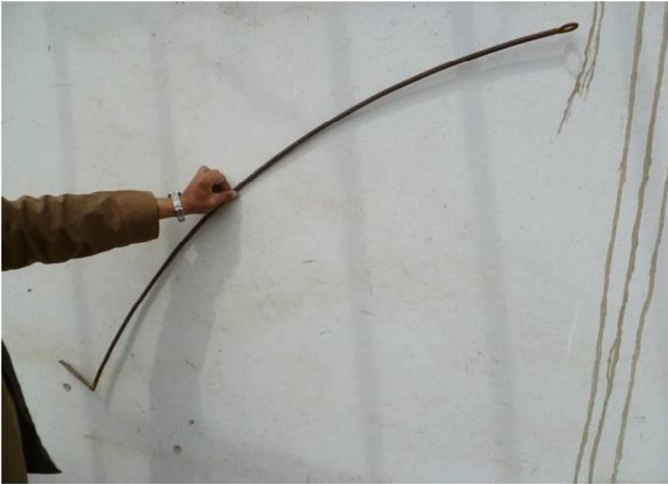
Figure 6.6.1: making shape of the dome using template
