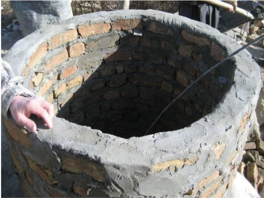
Figure 6.8.2: Inlet Tank during masonry construction.
