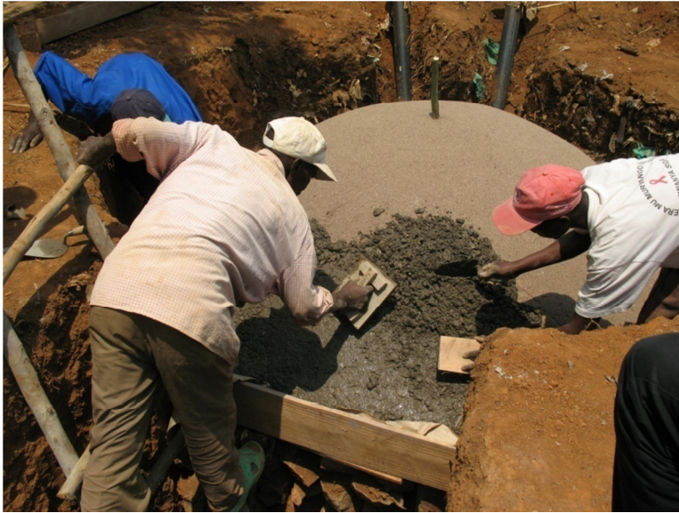
Fig 6.6.5 Plastering of digester and gas holder
