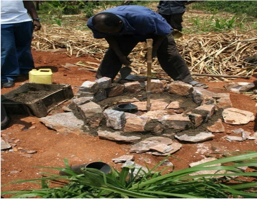
Fig 6.8.1 Inlet tank construction
