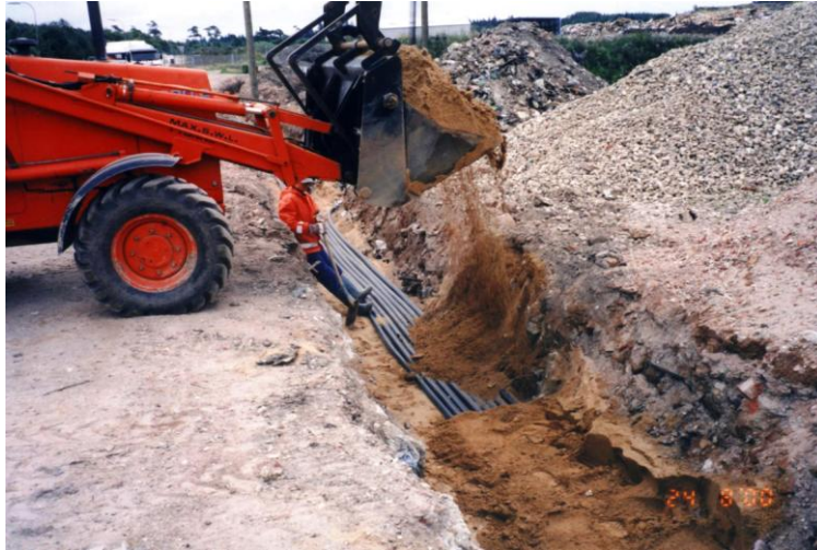
Illustration 12. Covering horizontal gas pipes for protection against frost
