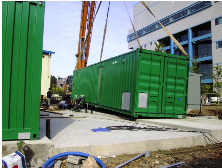
Illustration 13. Installation of a container with a compressor and gas cooling system
