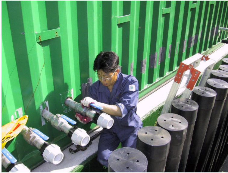
Illustration 14. Connection of gas pipes to a pump and regulation container
