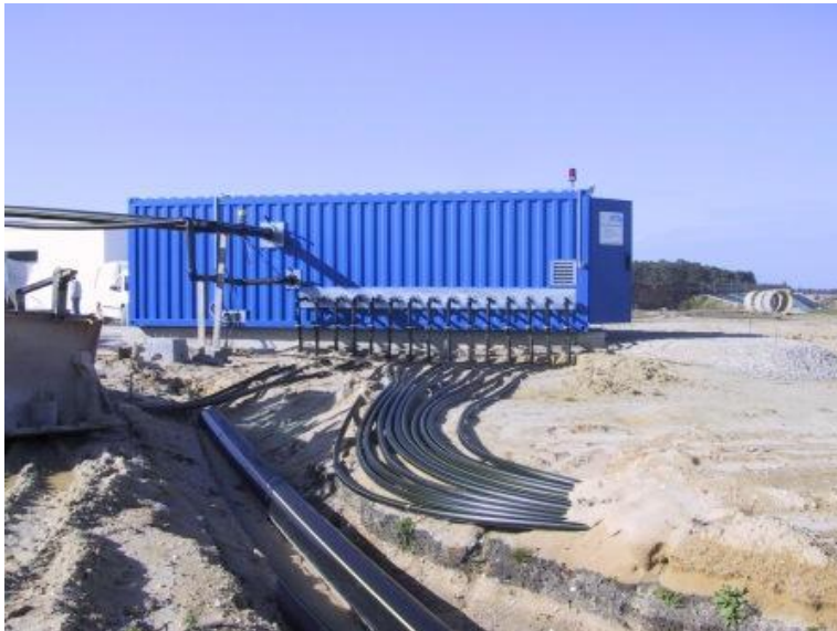
Illustration 15. Connection of gas pipes to a pump and regulation container
