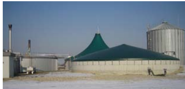
Photo 14: General view of a 1 MW el. energy crop co-digestion plant using two parallel digesters (left background) and a covered final digesterate storage tank (center foreground). Gas storage is integrated in digester 2 (background) and in the final storage tank (foreground), further storage capacity is provided in a dry gas storage tank (background right).
