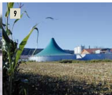
Photo 9: General view of a 2-step energy crop digestion plant with digester 1 (right) and combined gas collector and digester 2 (left)
