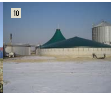
Photo 9: General view of a 2-step energy crop digestion plant with digester 1 (right) and combined gas collector and digester 2 (left)
