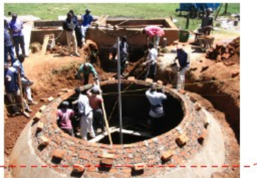
Figure 7: Construction of the dome.
