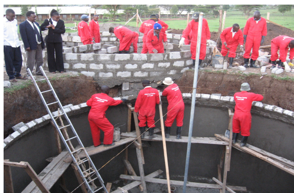
Figure 6: Inside of round-wall plastered with a smooth layer of cement mortar.
