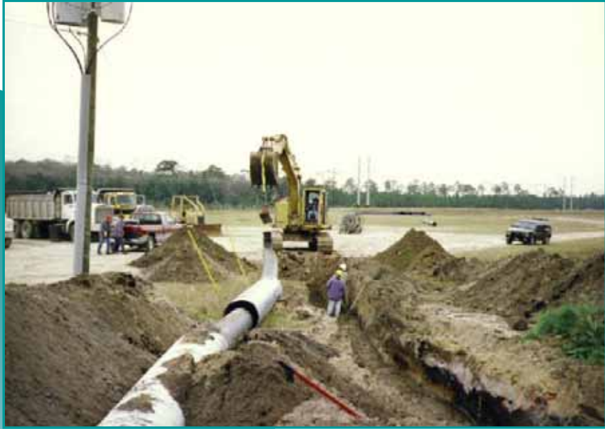
LFG header roadway crossings
