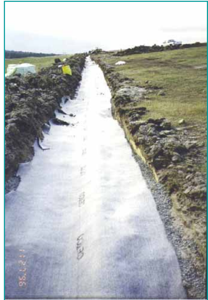
Geosynthetic liner over trench
