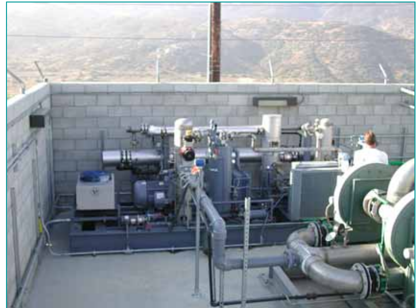
Blower and Compressor Skid
