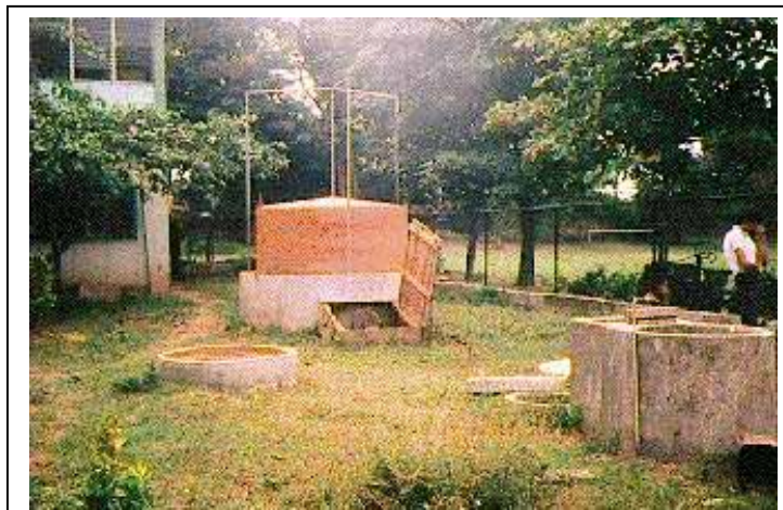
Figure 18: Biogas plant with separate gasholder in Nicaragua
