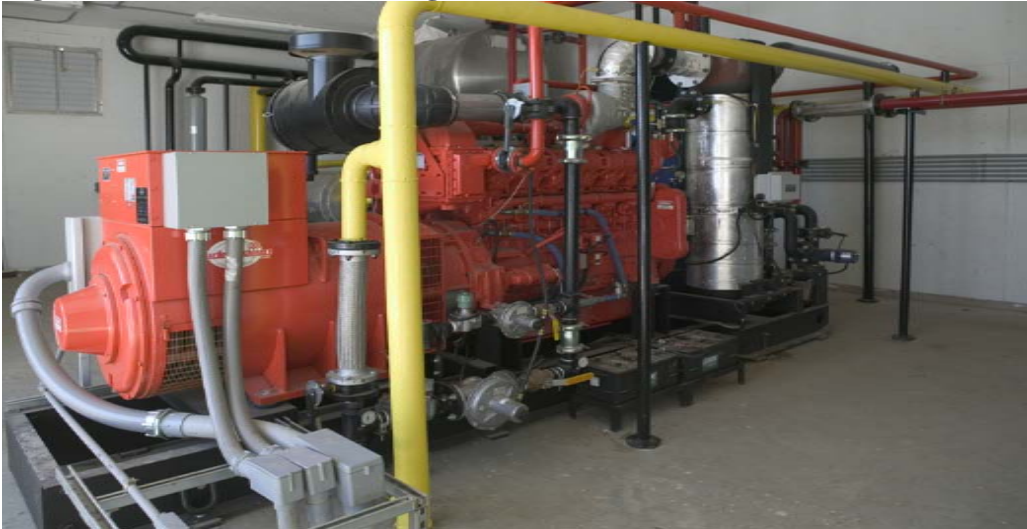
Figure 7 – Guascor 300 kW Engine Generator Set
