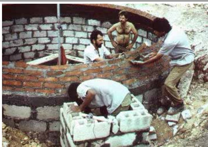
Figure 17: Construction of the dome for a 30 m 3 digester in Cuba Photo: Krämer (TBW)
