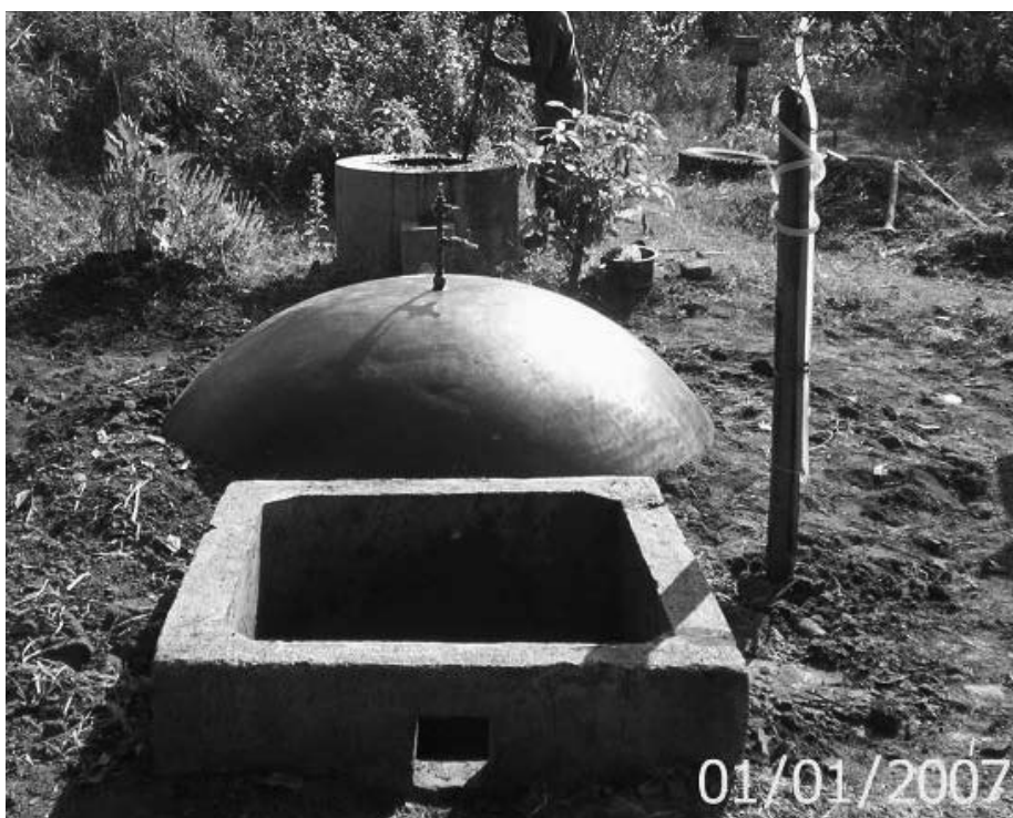
Figure 3. Biogas plant during construction (Photo: CV Krishna)
