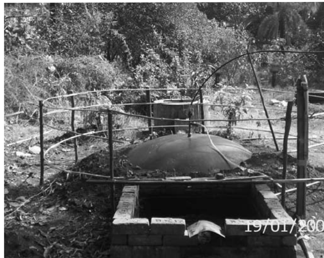
Figure 2. Finished Biogas plant with PE Dome (Photo: CV Krishna)
