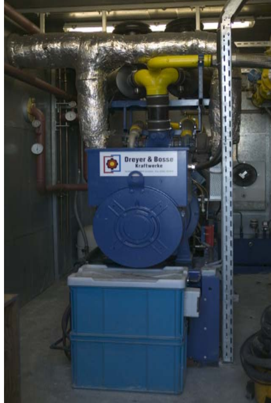
Figure 43 – Suring Engine Generator Set
