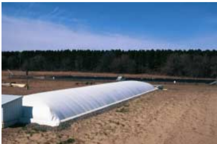
Anaerobic plug-flow digester. Haubenschild Farms, Inc.
