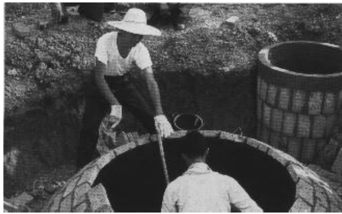
Figure 6: Installation of a Shanghai fixed-dome system near Shanghai, PR China
