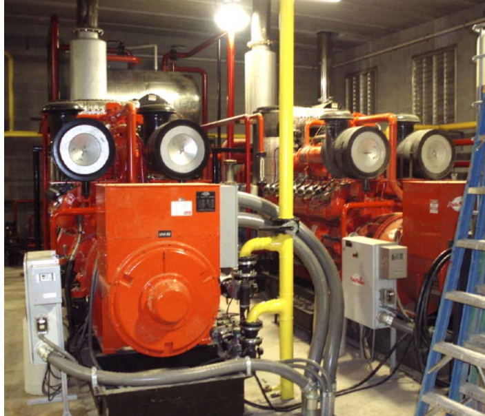
Figure 29 – Holsum Engine Generator Sets at Elm Road
