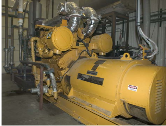
Figure 19 – Double S Dairy Engine Generator Set
