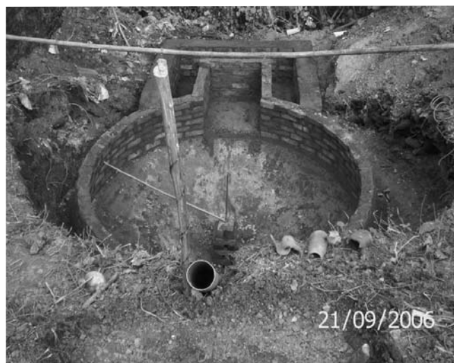
Figure 1. Digester wall construction (Photo: CV Krishna)
