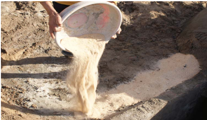
Figure: 16.1 sand filling to raise the area to required height
