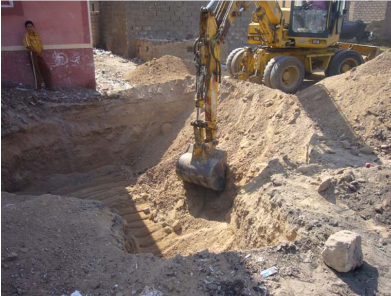
Figure: 6.1 Excavation of a pit for plant installation using machine
