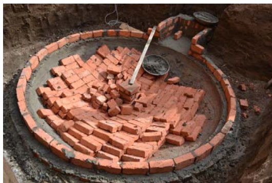
Figure: 11.1 starting construction of the digester
