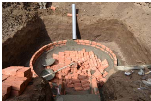
Figure: 12.1 Placing of inlet pipe 1
