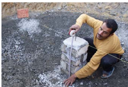
Figure: 8.1 Construction of centre pillar
