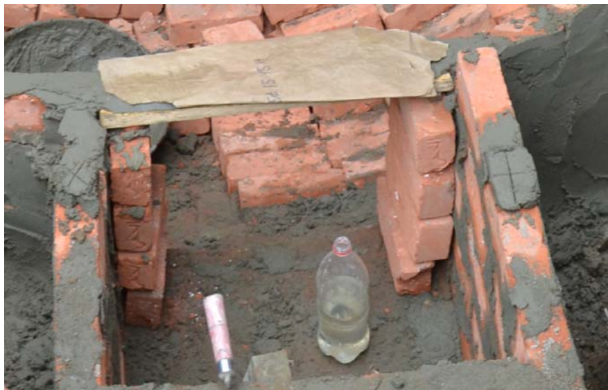
Figure: 14.1 Support plank for box tank ceiling layer
