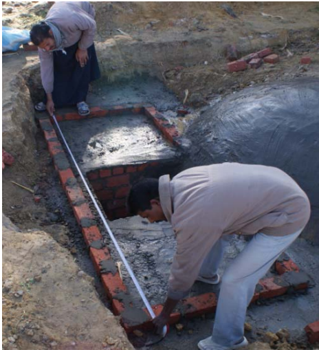
Figure: 17.1 First layer of bricks
