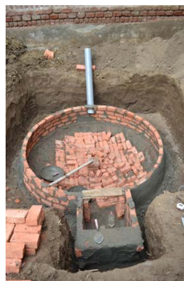
Figure: 12.4 Fixing of inlet pipe lower than the slurry flow gate height
