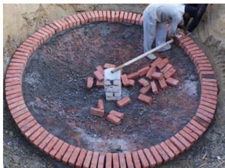
Figure: 10.1 Laying of 1 st layer of bricks
