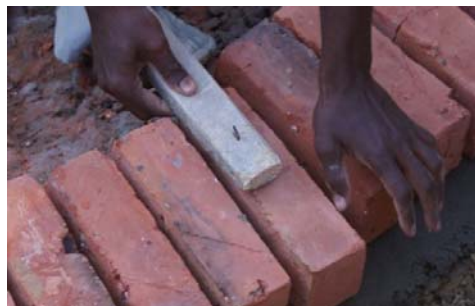
Figure 10.2: Spacing first layer of bricks
