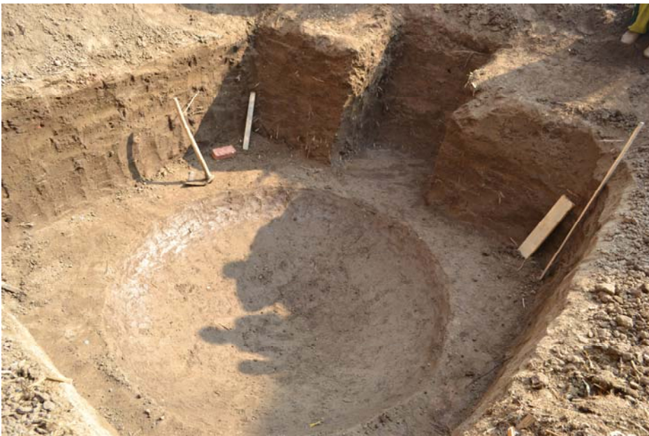
Figure: 6.2 A trimmed pit ready for bed concrete
