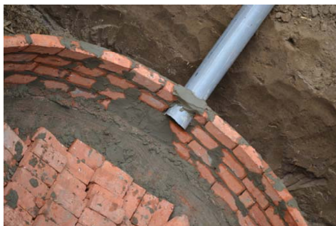
Figure: 12.3 Fixing of inlet pipe
