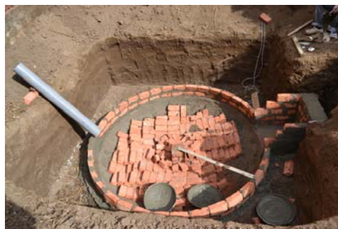
Figure: 12.2. Placing of inlet pipe
