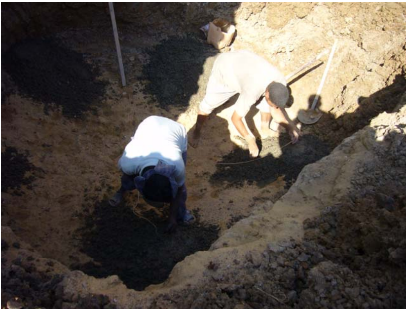
Figure: 7.1 maintain the level of bed concrete all the round using plastic tube filled with water
