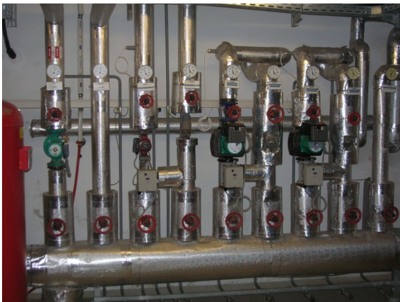
Figure 23: Heat distribution in biogas plant. Professional concepts may utilise a large proportion of heat produced. Photo: MEP.
