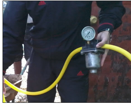
Fig. 2. Biogas Sampling Line.
