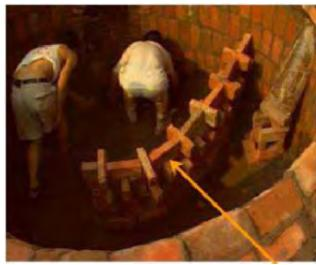
**Figure 3:** Internal baffle wall
