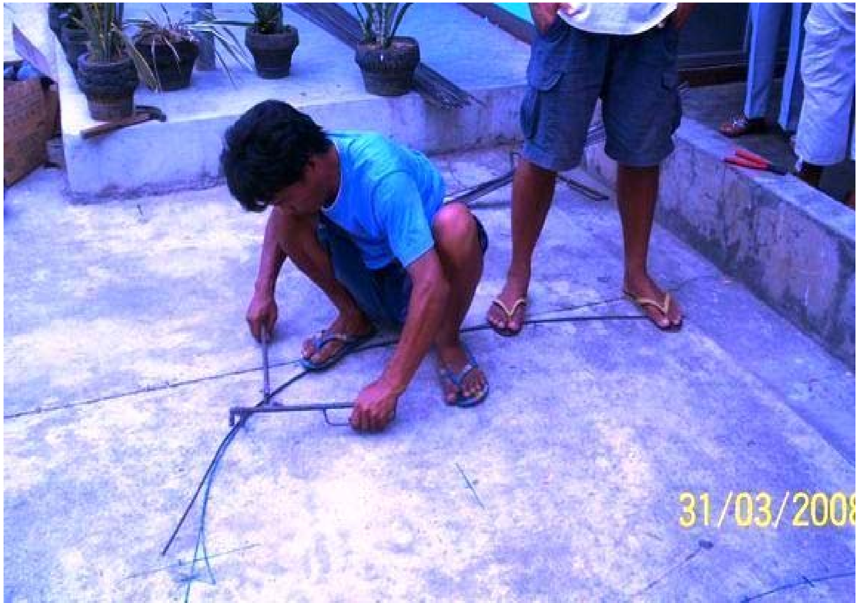
Bending the mold rebars
