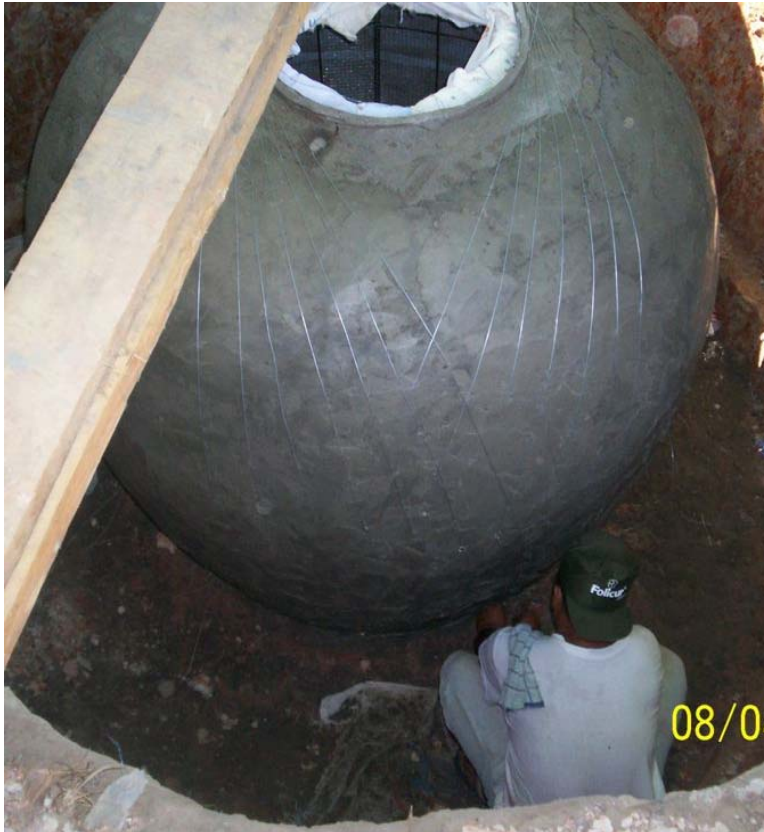
Vertical wires reinforcement for the digester
