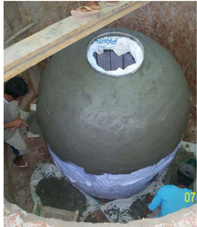
First mortar coating of the digester.
