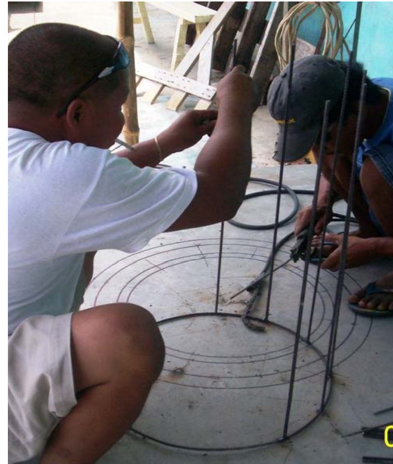
Walling-in culvert mold welding
