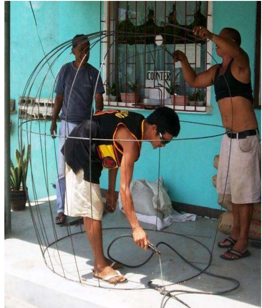
Digester mold welding
