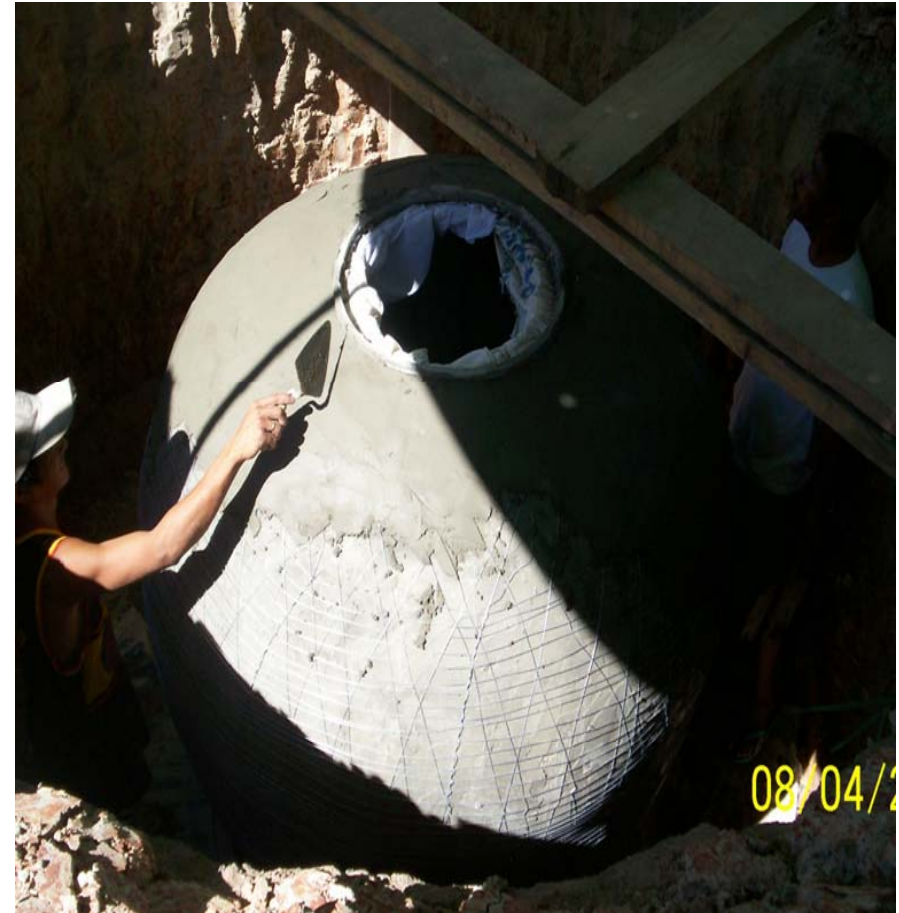
After the horizontal wiring is laid, a finishing mortar coat.
